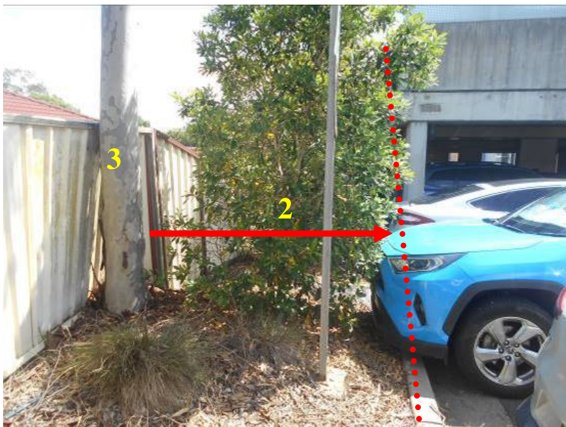
Figure 5 – showing the location of Trees 2 & 3 inside the existing garden bed. The 2 nd storey car park will extend to the east quadrant past Trees 2 & 3. The proposed car park will be located 2.15 metres to the trunk of Tree 3. This species
