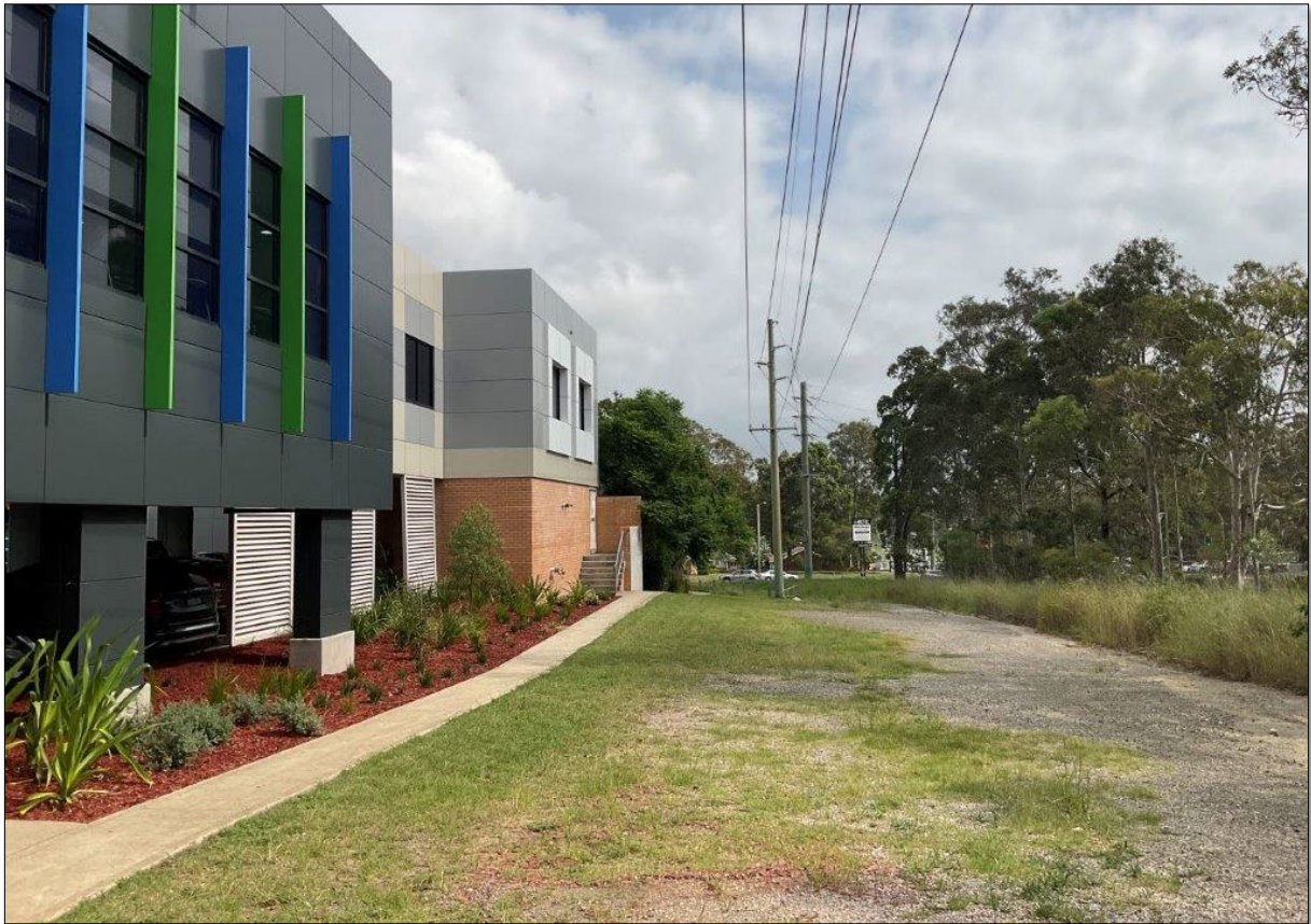
Plate 11: The fire trail adjoining the northern elevation is roughly formed and unsealed, but a minimum 6m wide in most areas
