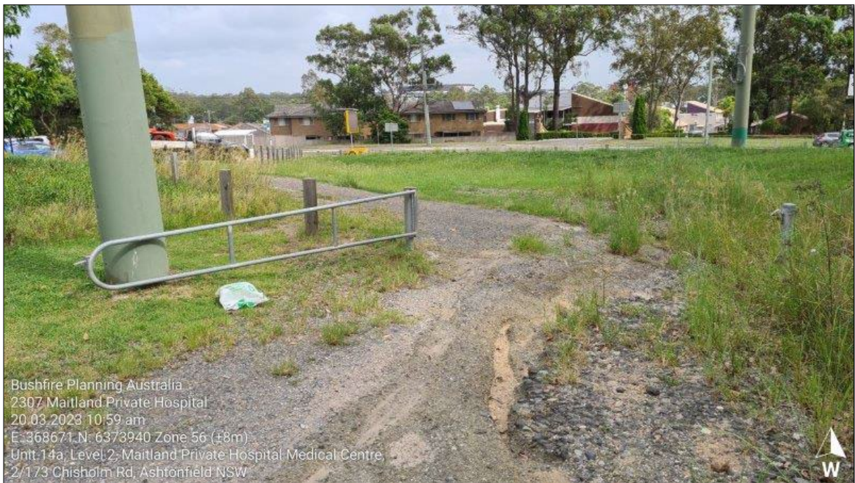
Plate 7: Unauthorised access to the northern access track is able to prevented by a lockable gate
