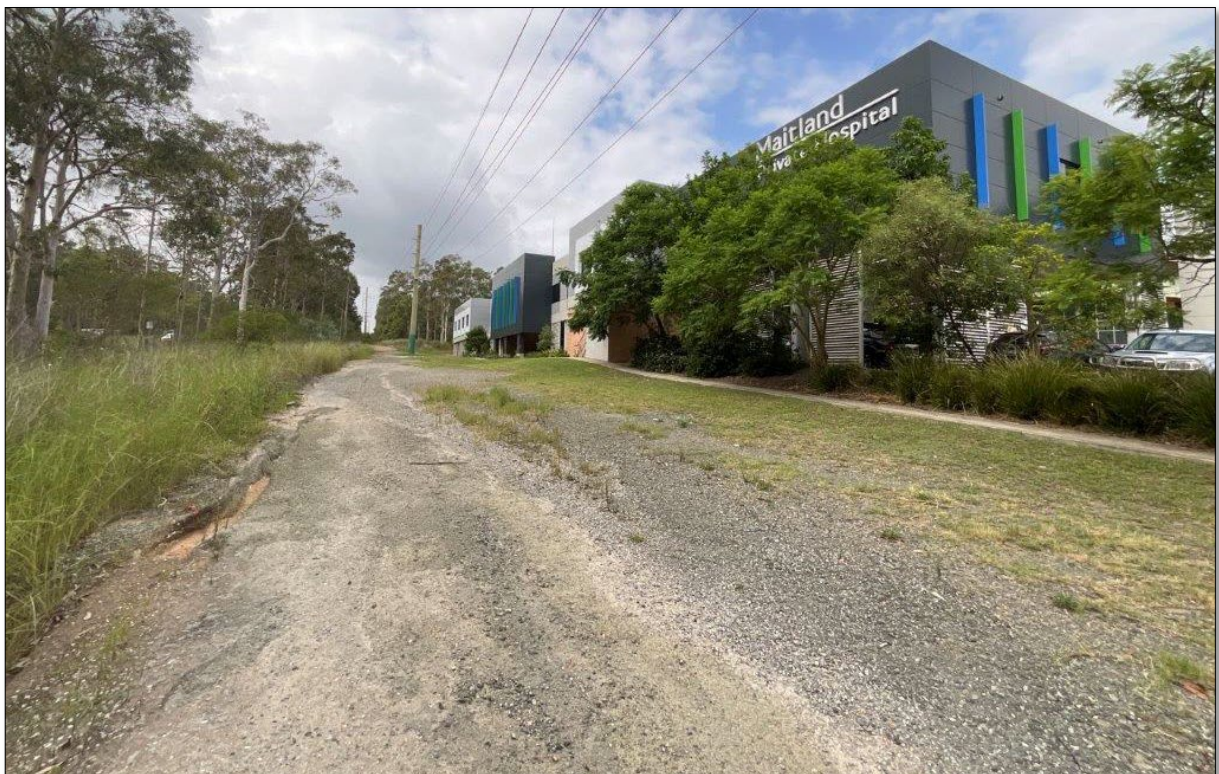
Plate 12: The fire trail adjoining the site is serviceable for use by emergency services
