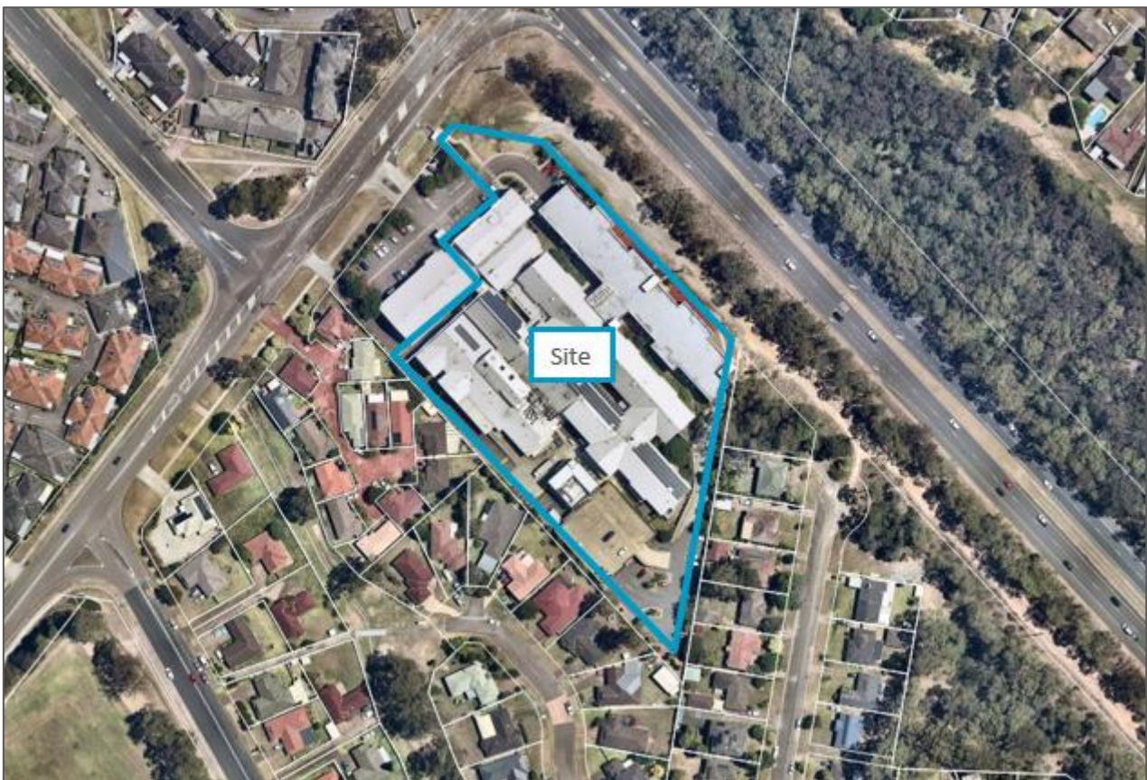
Figure 1 Site Aerial (Source: SixMaps)
