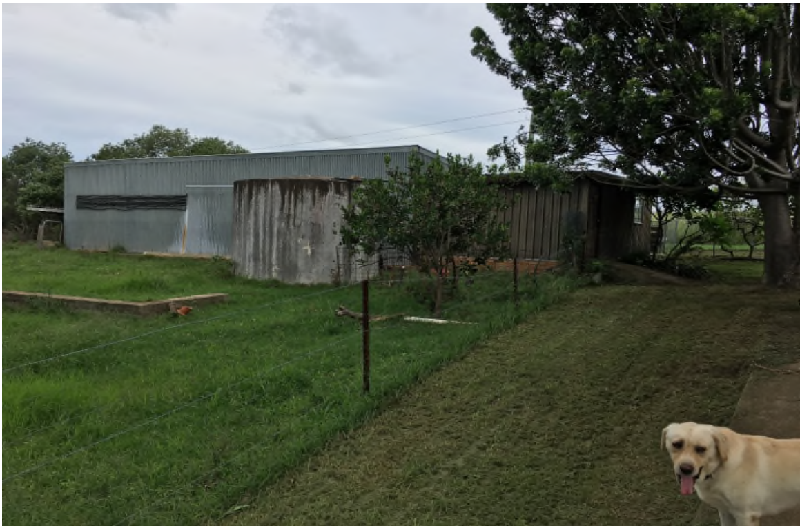
Photograph 4: Shed and water tank on Lot 2
