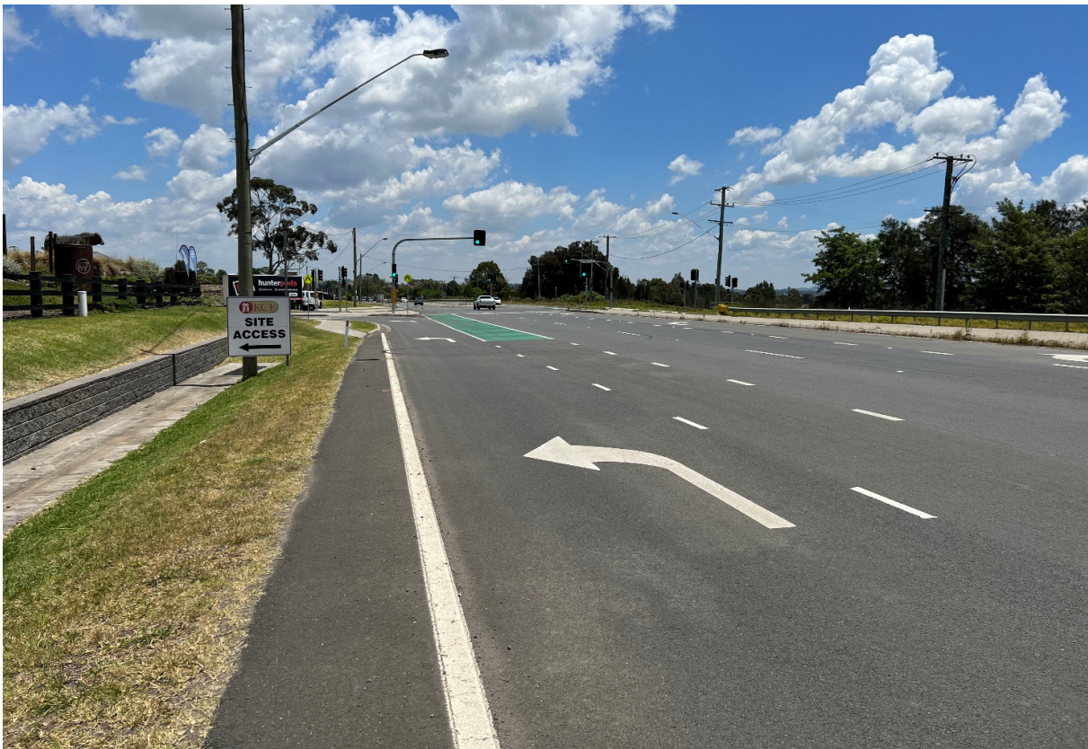
Photograph 2 – New England Highway / Springfield Drive signalised intersection.
