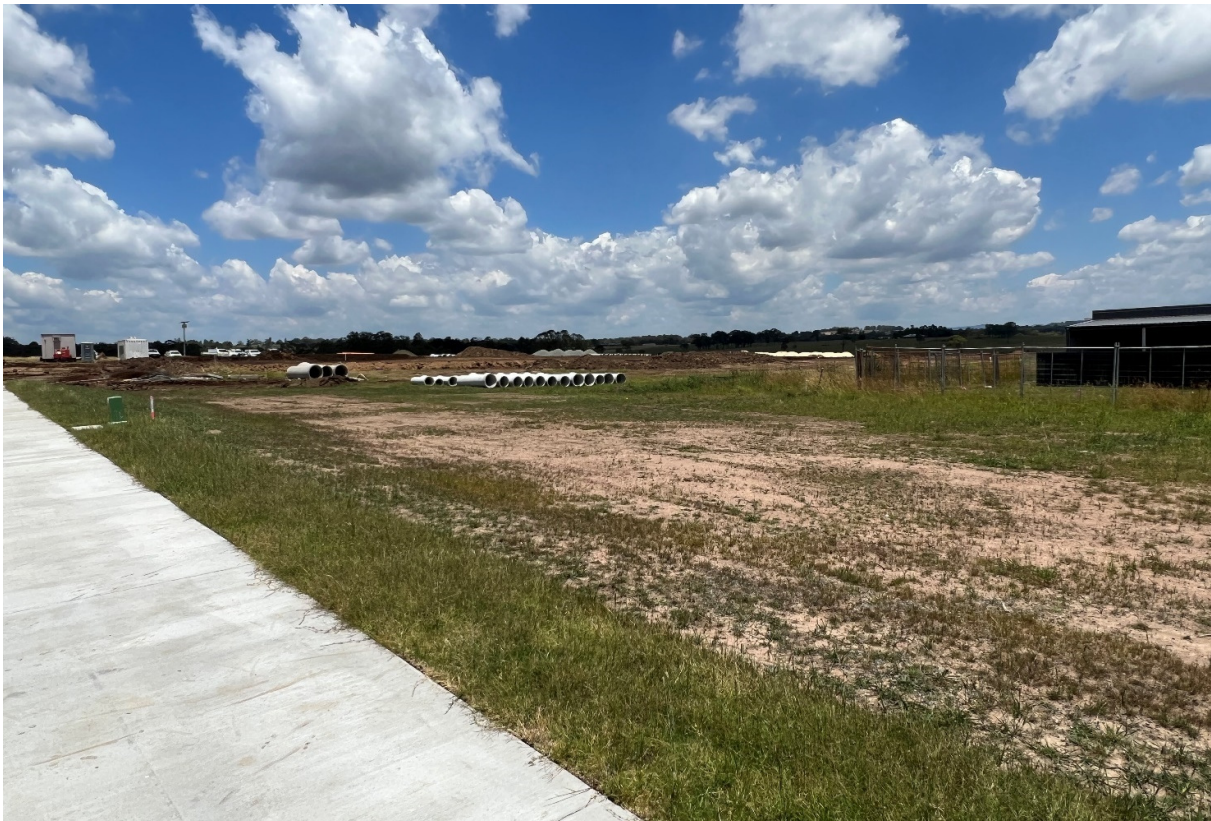
Photograph 1 – Existing site conditions.
