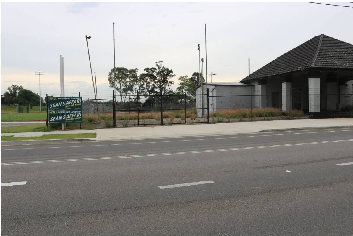
Photograph 2 – Existing western vehicular access.
