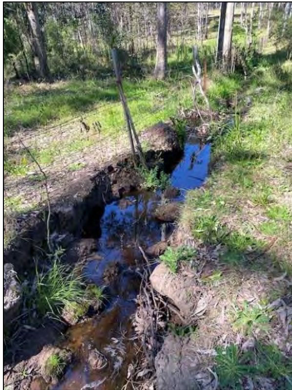
Below: Drainage line from large dam
