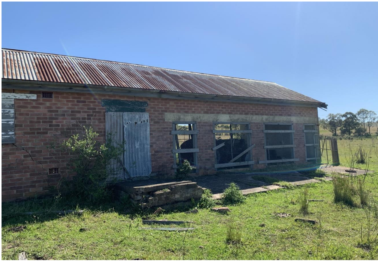
Photograph 7 - Showing outside of brick and metal clad barn.
