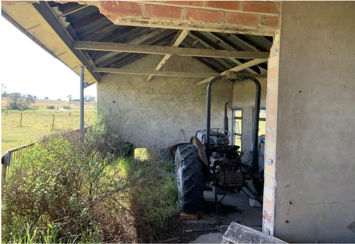
Photograph 9 - Showing tractor on concrete flooring and overgrown weeds.
