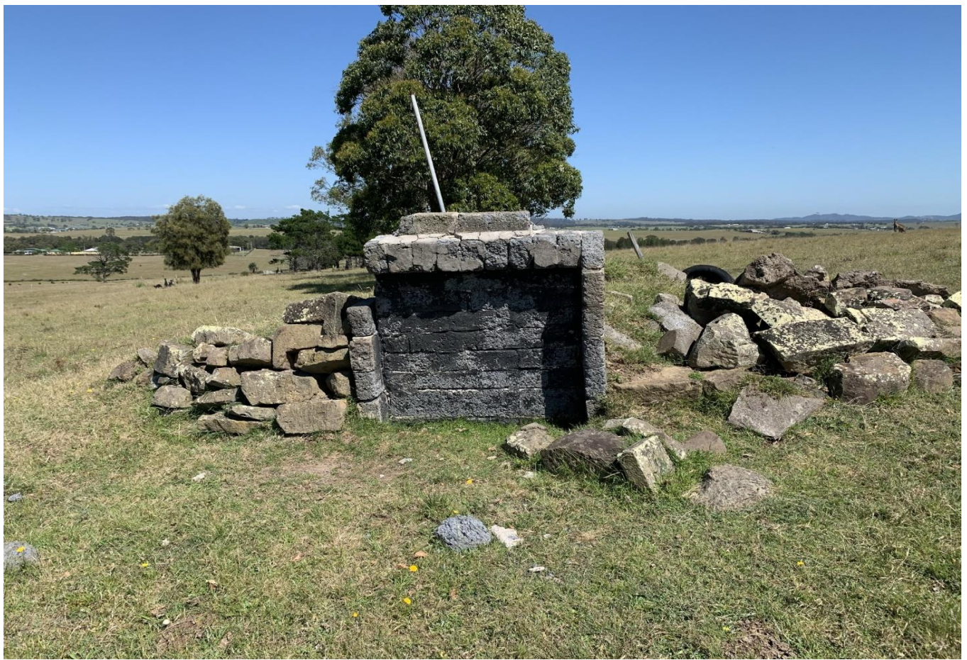
Photograph 5 - Showing Stockpile (SP1) of house rubble in central portion of site.
