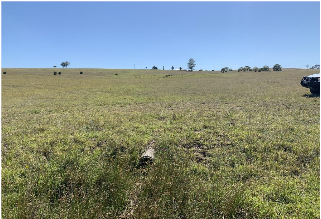
Photograph 6 - Showing exposed pipe in fill.
