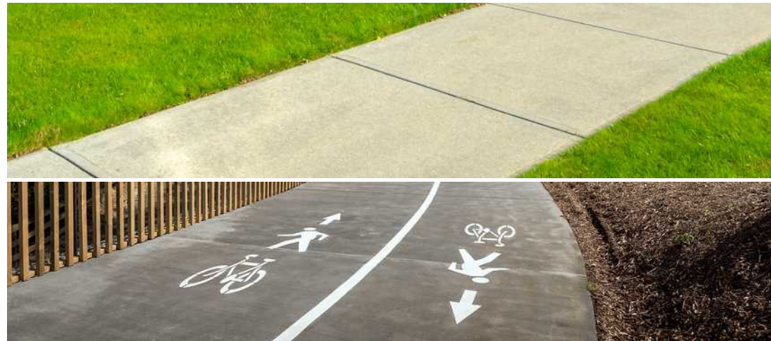
PATHS: BROOM-FINISH STANDARD CONCRETE TO 1.5m AND 2.5M PATHS THERMOPLASTIC MARKINGS SHARED-USED PATH NETWORK
