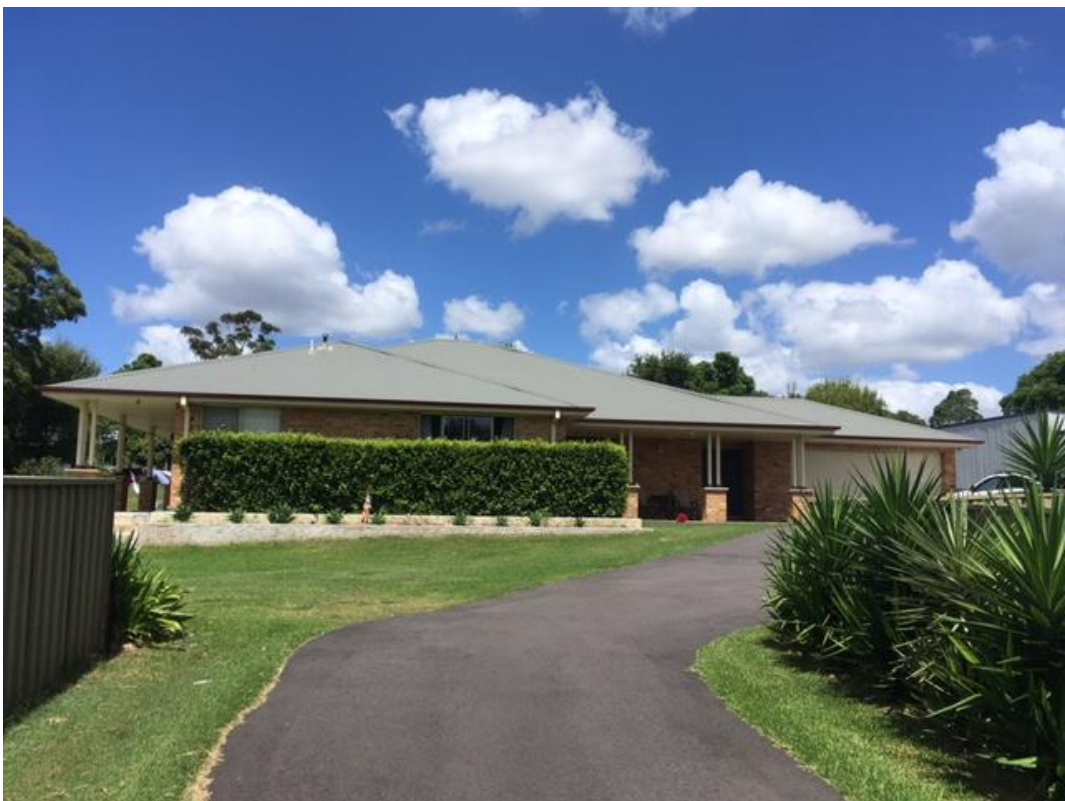
Figure 7 – Photo of existing dwelling at 23A Robert Street Tenambit – to be retained
