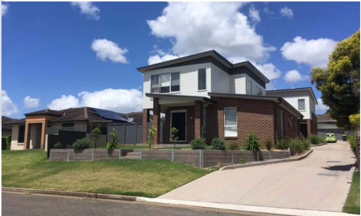
Figure 13 – Photo of recently constructed two storey units at Crawford Avenue Tenambit
