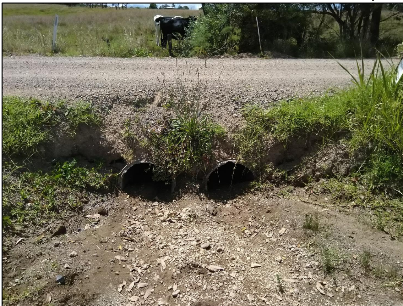
Figure 8 - Circular culverts beneath Wyndella Road. (Looking upstream)
