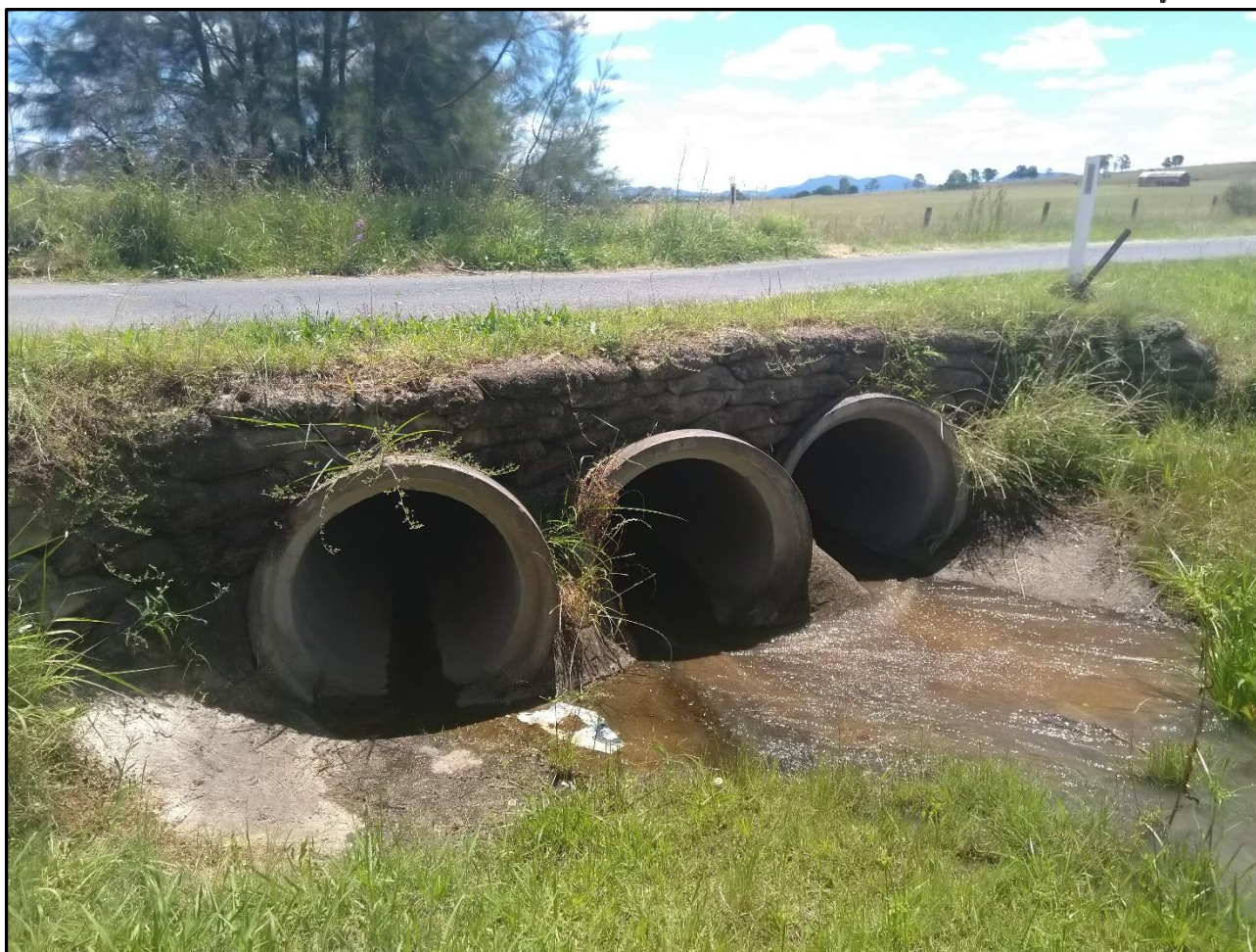
Figure 9 - Circular culverts beneath Wyndella Road. (Looking downstream)
