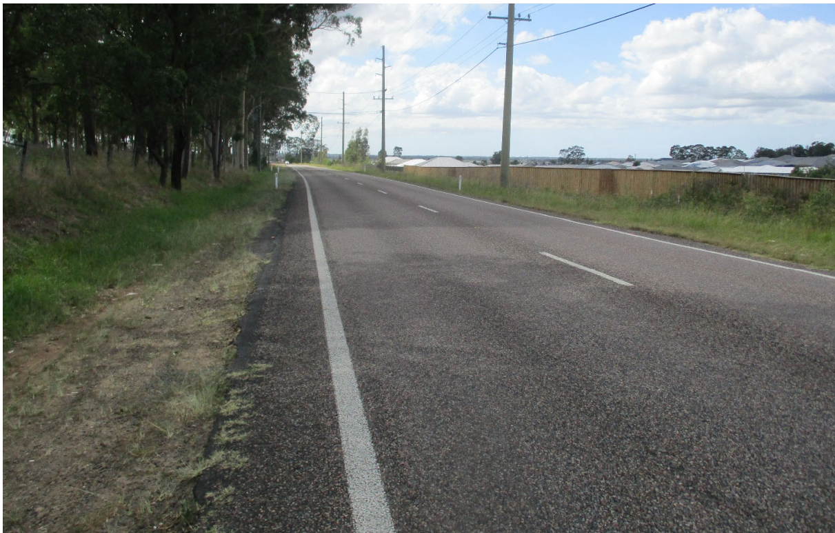
Photograph 3 – Raymond Terrace Road along site frontage.
