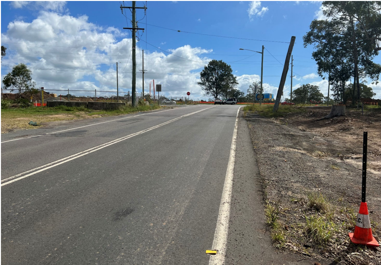
Photograph 5 – Raymond Terrace Road / Government Road upgrade under construction.
