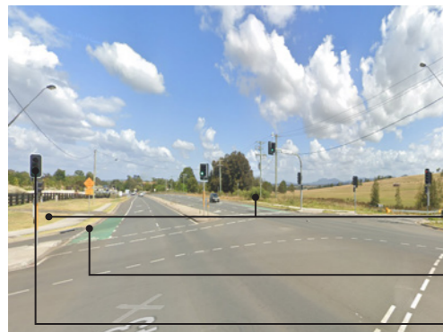
1- View of new intersection / site access
