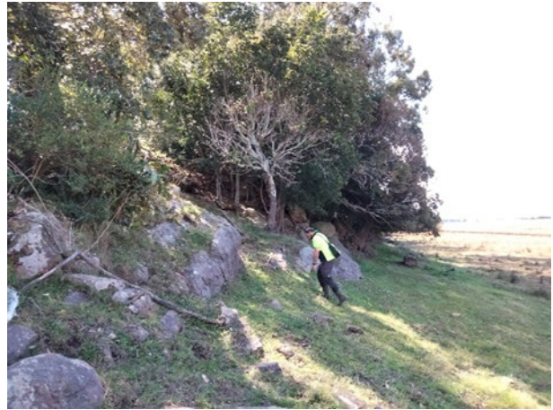
Plate 6: Base of sandstone ledges and boulders in south of survey unit, facing north-east
