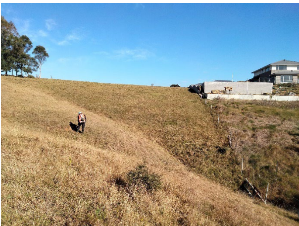
Plate 9: View over developing gully on northward slopes, facing west
