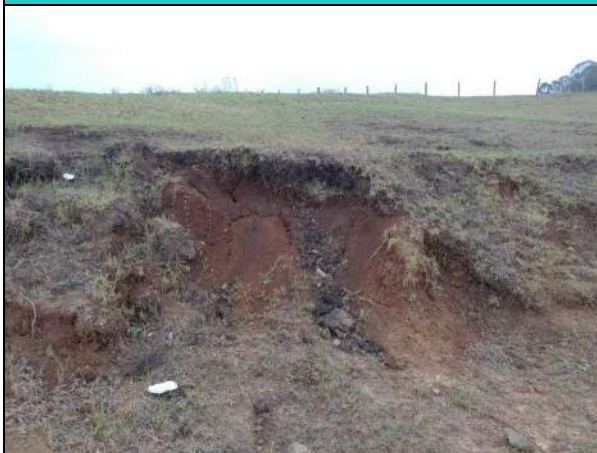
Photograph 11: Dam wall (North Elevation)
