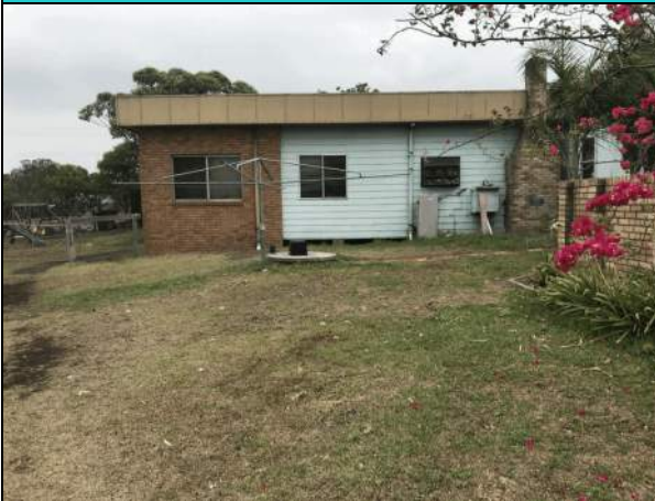
Photograph 3: Rear Dwelling Elevation
