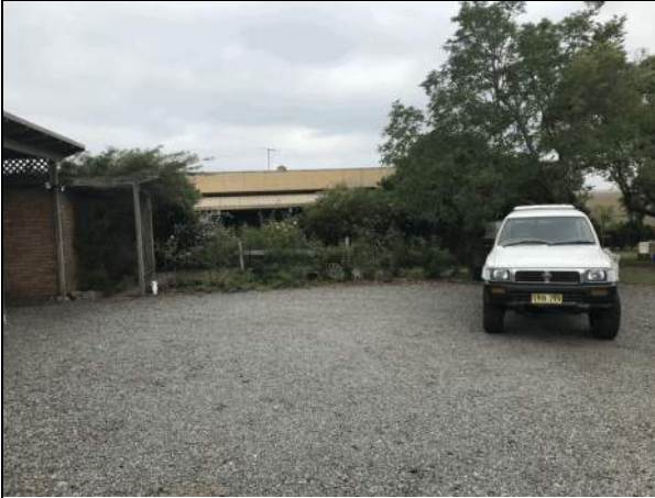
Photograph 1: Front Elevation of Dwelling.
