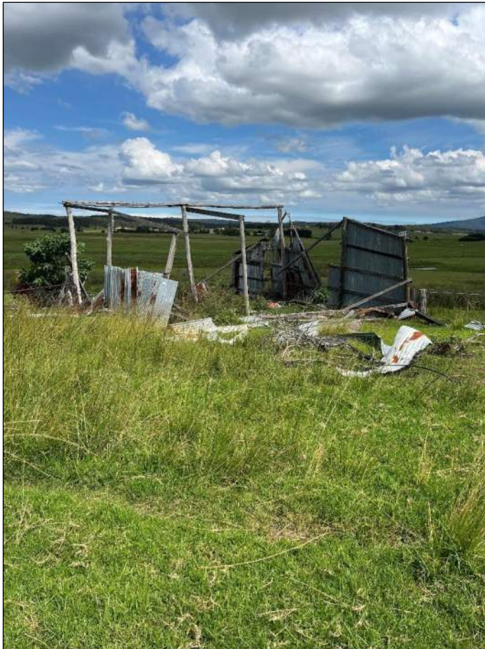
Figure 18: Building materials, remnant structure and uneven ground in the central-southern portion of the site, looking south-east
