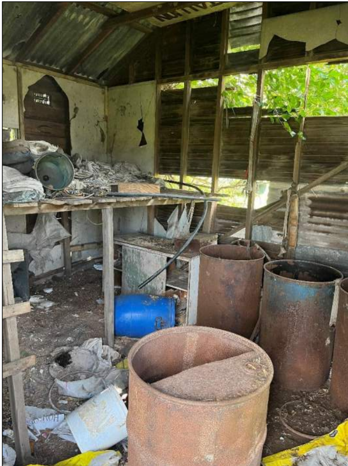
Figure 22: Oil/fuel barrels within the former dairy structure in the central-southern portion of the site
