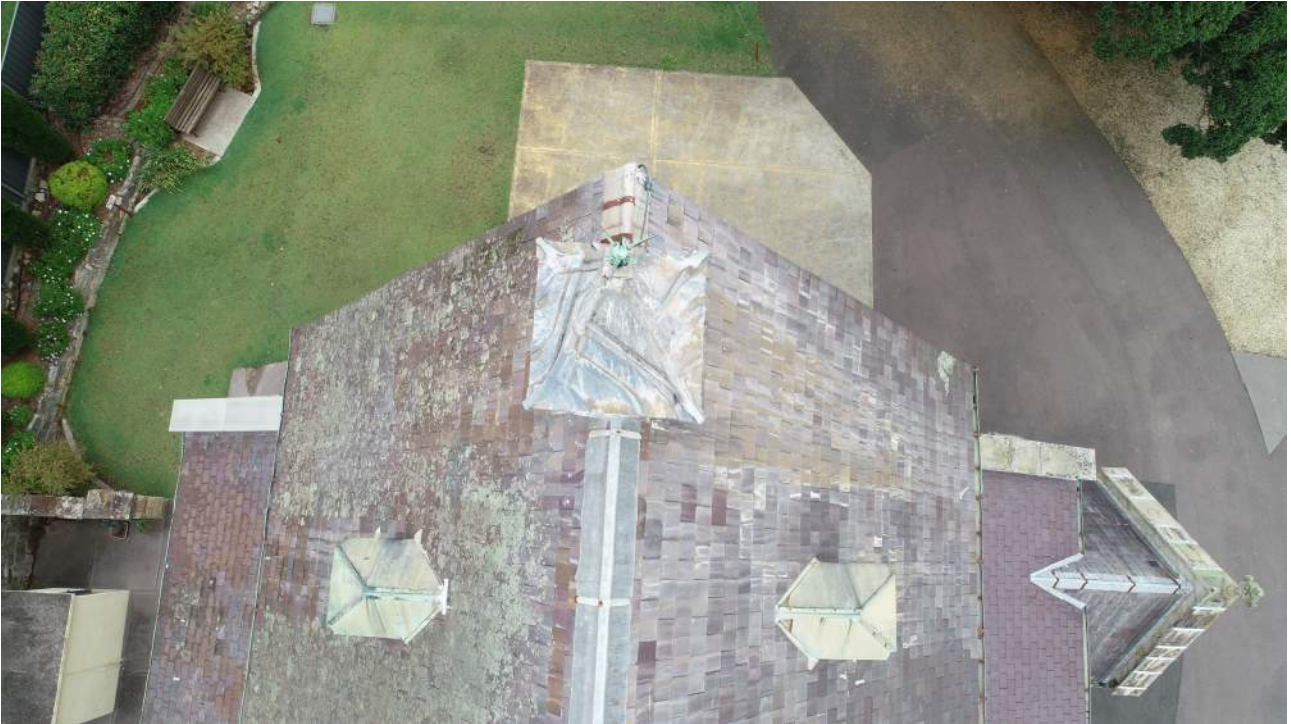
Figure 35 Aerial view of bellcote to western apex with rolled lead sheeting and copper lightning rod. source: iScope Consultants, March 2021.
