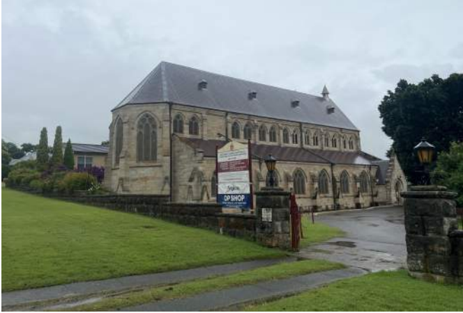
Figure 15 View of church from William Street with vehicle access provided. source: Heritas, 2022.
