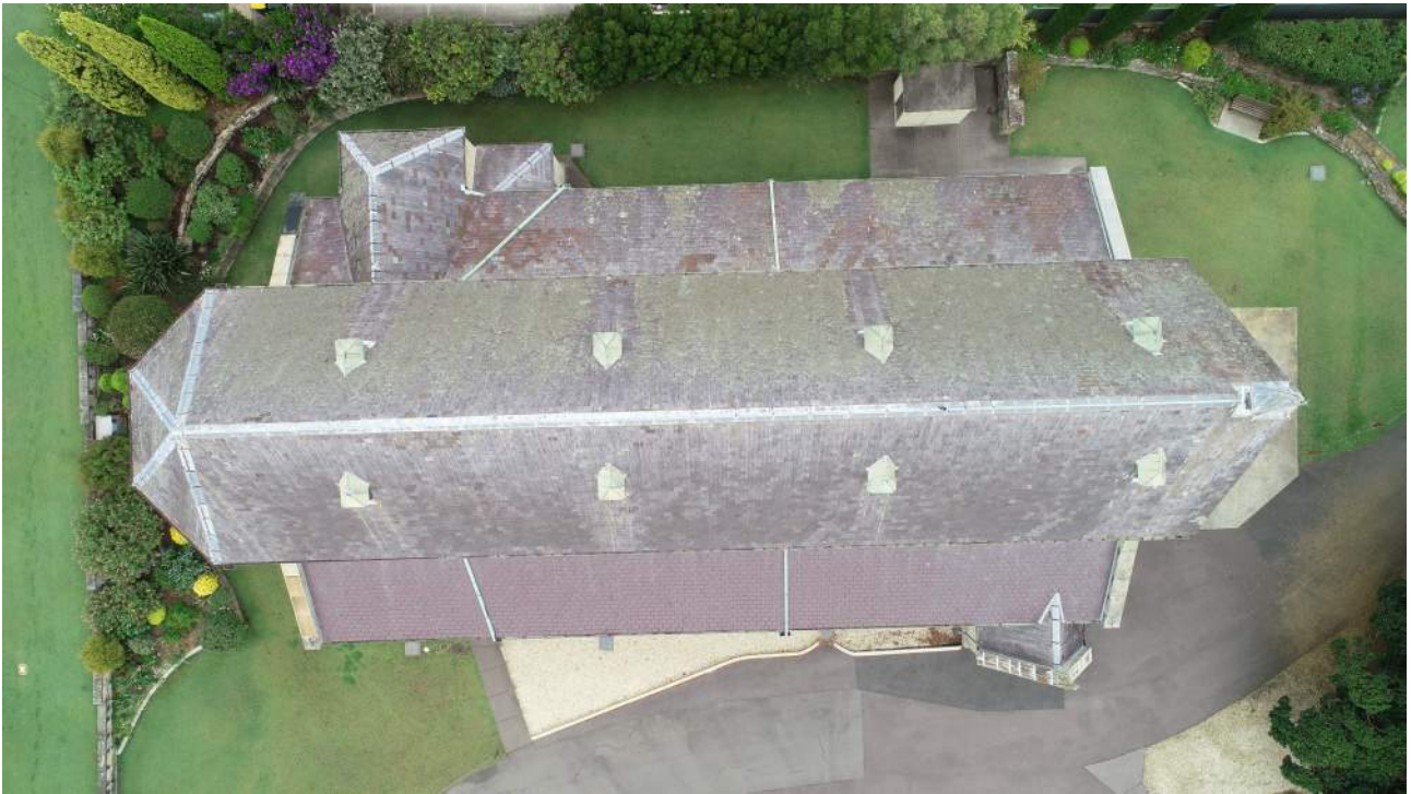
Figure 27 Aerial view of slate roof to church. source: iScope Consultants, March 2021.
