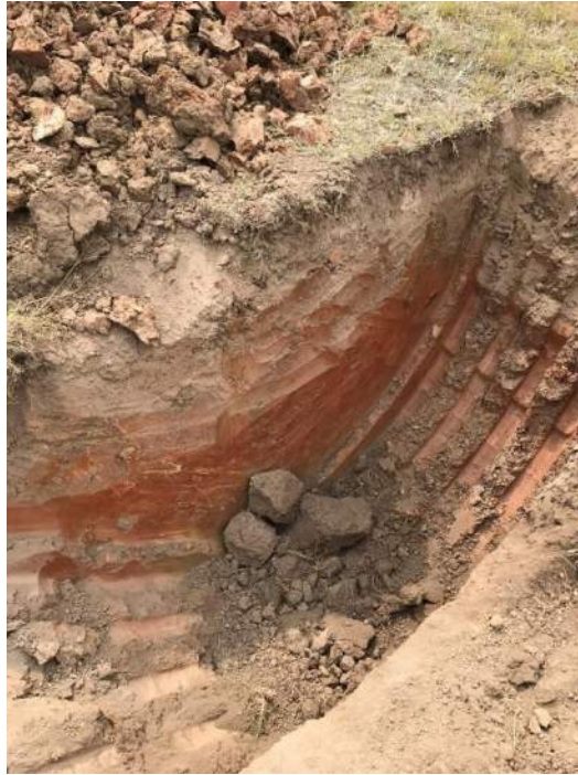
Plate 15 – Typical sub surface conditions observed across the Site. Date: 8/5/2020
