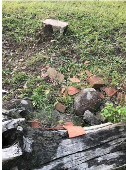
Plate 9 – Buried concrete and brick located between Dam 02 and Dam 03.
