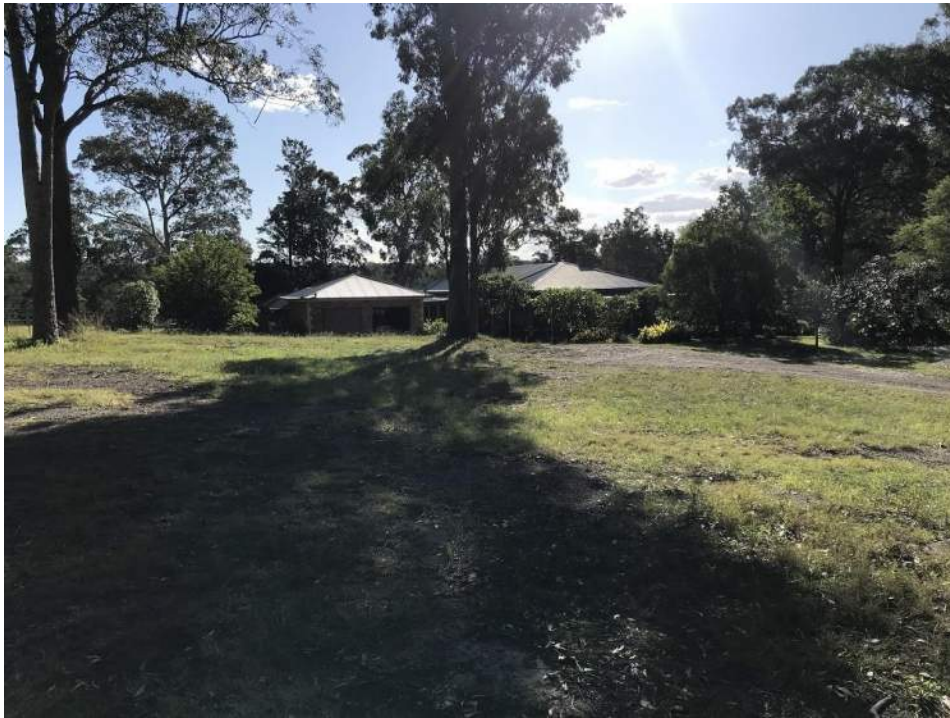
Plate 1 – Brick residential dwelling located in the northern portion of the Site. Date: 8/5/2020
