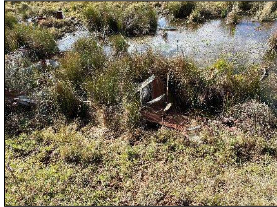
Plate 2: Segment ID 1.1 Facing east across dam.
