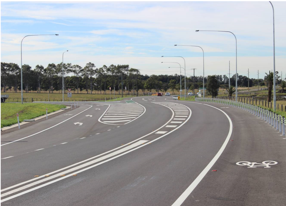
Photograph 3 – Raymond Terrace Road looking east ( McFarlanes Road on left)
