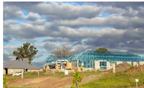
Image 22 Construction associated with R1 General Residential zone
