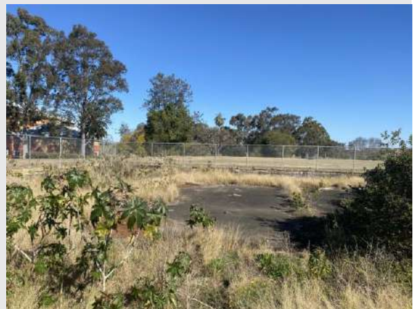
Photograph 10 – A filter bed at southern end of former water treatment area
