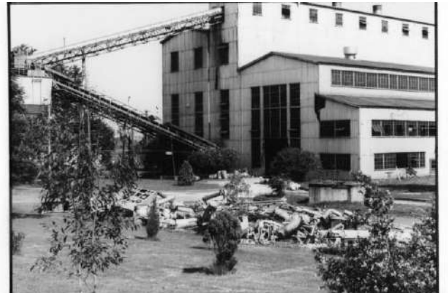
Power station demolition, January 1978
