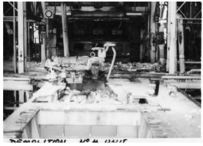
Power station demolition, January 1978
