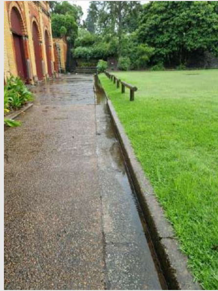
Photograph 2 – Heritage kerbs east of pump house
