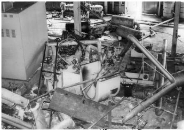
Power station demolition, January 1978
