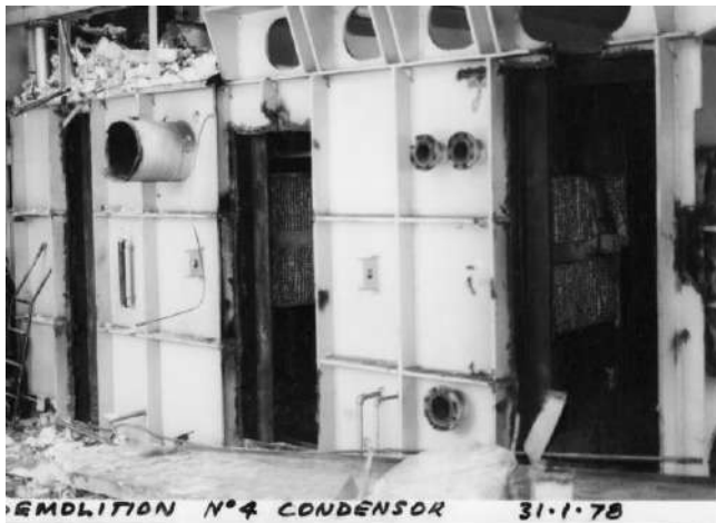
Power station demolition, January 1978
