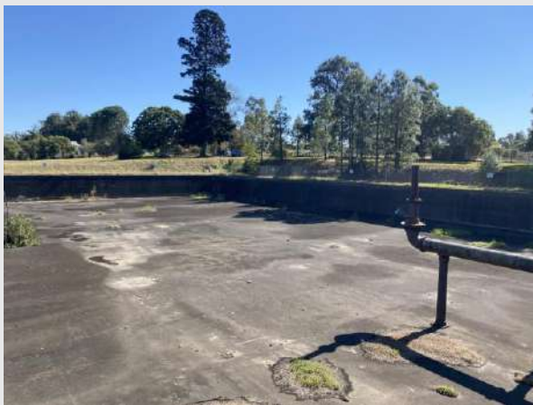
Photograph 9 – Settling tank, northern end of former water treatment area
