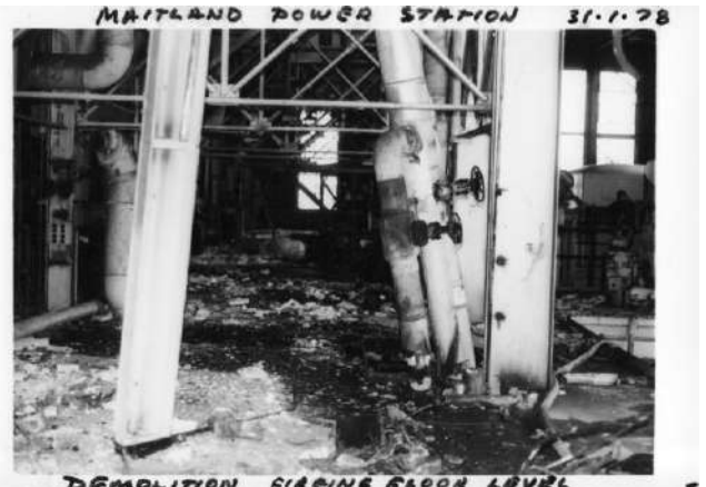
Power station demolition, January 1978
