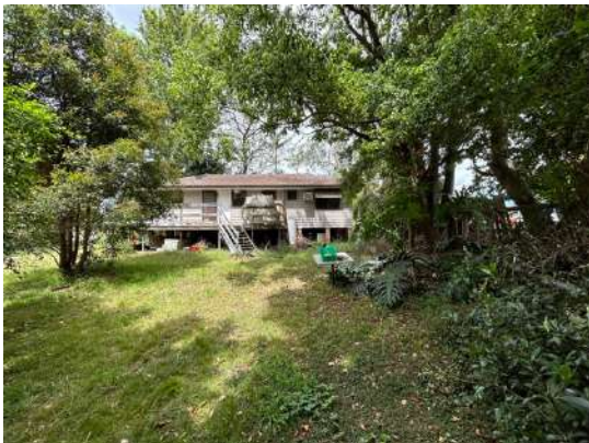
The rear of the dwelling presenting towards the railway line.
