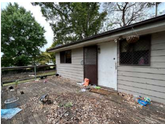
Rear deck area showing fibre-cement weatherboard cladding and aluminium windows.
