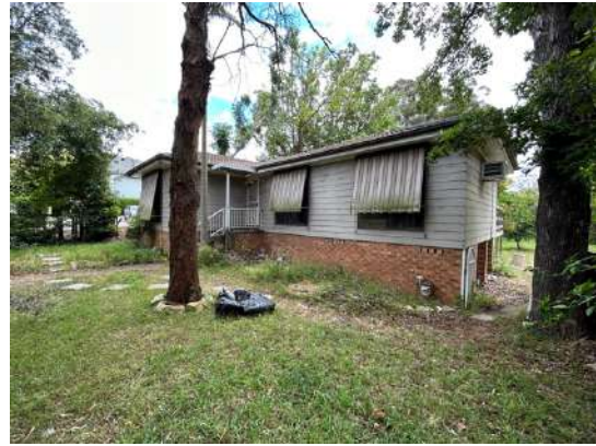
Front elevation showing brick subfloor with fibre-cement weatherboard dwelling over.
