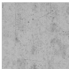
CONCRETE HARDSTAND AREAS
