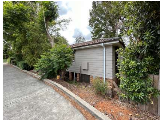
North-western elevation as viewed from the adjacent hotel.
