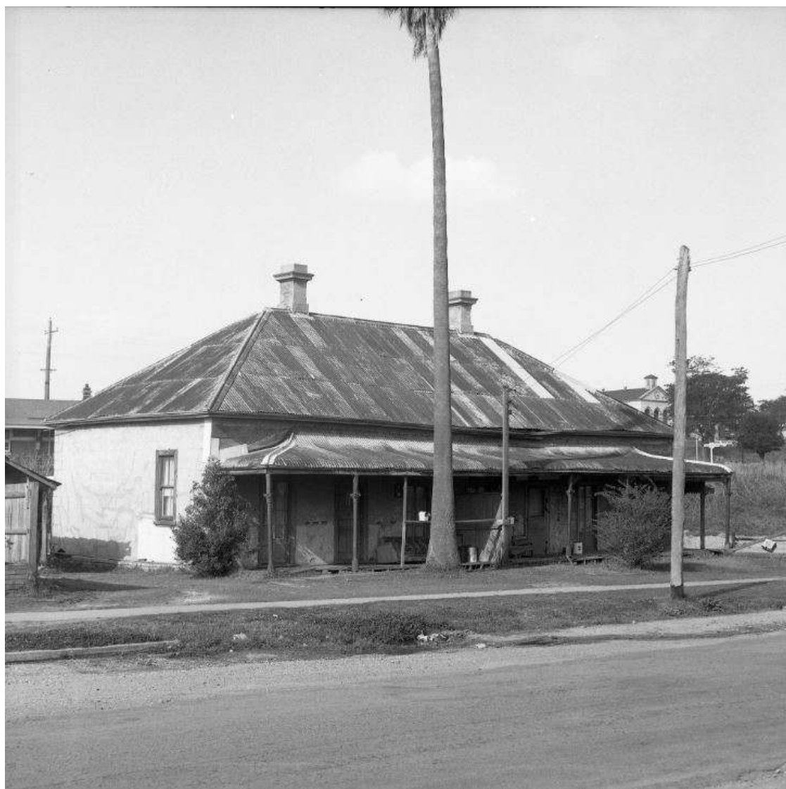
Figure 10 Old house no. 12 Day Street, opposite Roseneath, East Maitland, NSW The East Maitland Courthouse is visible in the background to image right and East Maitland Railway Station in the background to image left.
