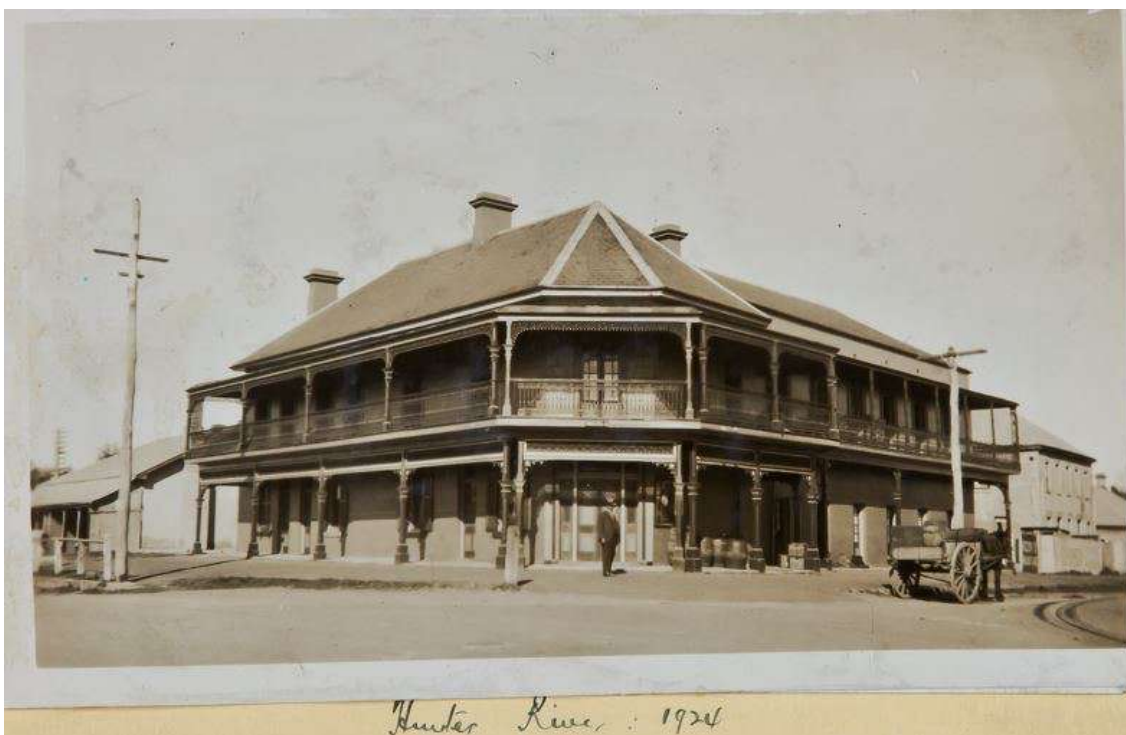
Figure 6 Hunter River Hotel, Melbourne Street, East Maitland Former Maitland Wine Vaults 1924
