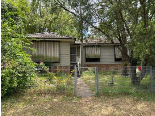
The front of the dwelling presenting to Day Street. Overall Condition: Poor
