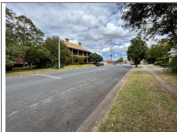
Looking from the front boundary of the site towards the north along Day Street. Roseneath is the dominant element to image centre.
