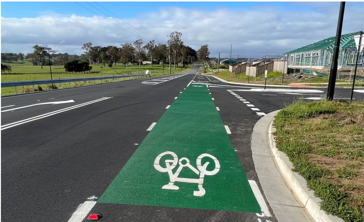
Photograph 7 – McFarlanes Road / Settlers Boulevard intersection.
