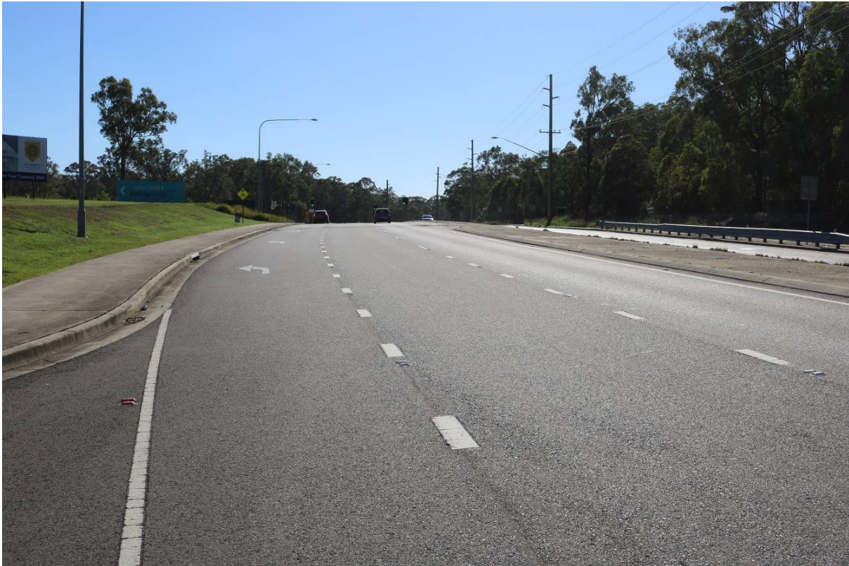
Photograph 3 – Raymond Terrace Road at Settler's Boulevard intersection.
