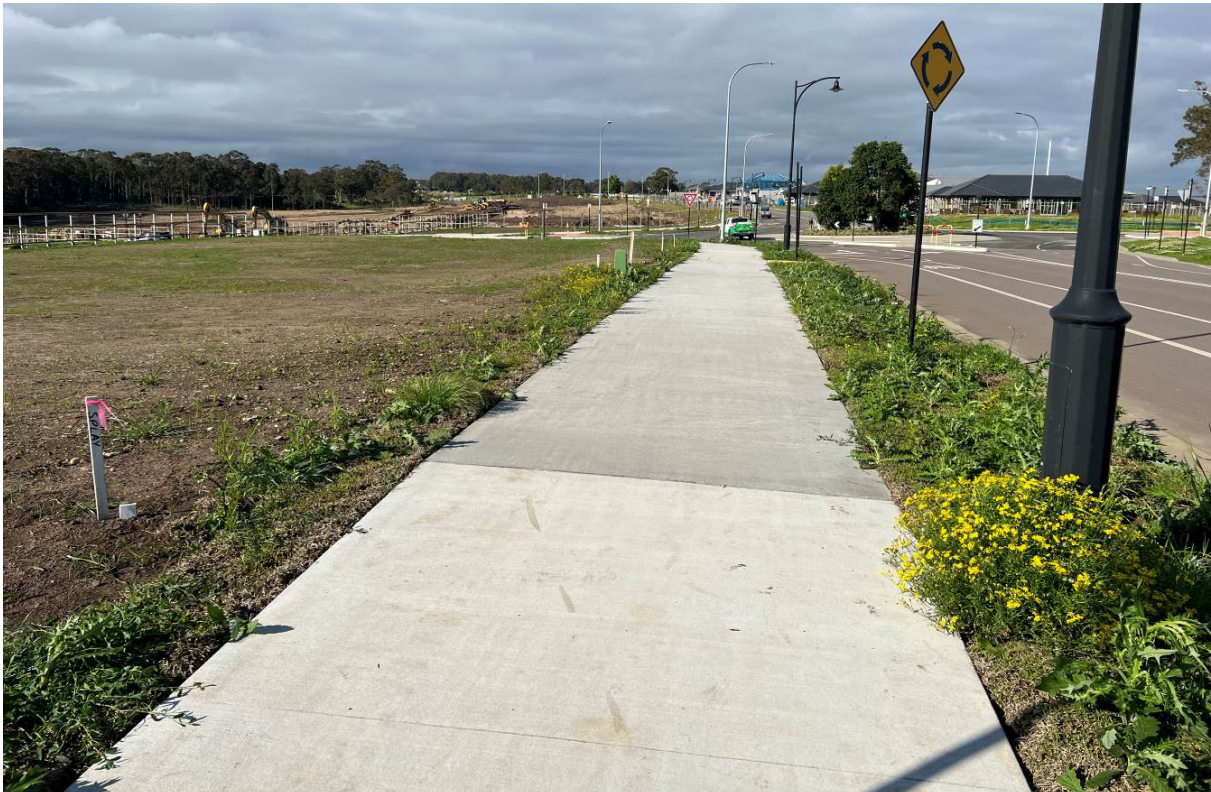
Photograph 2 – Settlers Boulevard / Caldera Street / Steamcruiser Drive roundabout.
