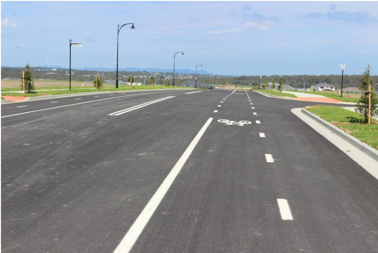
Photograph 4 – Dragonfly Drive near the site.
