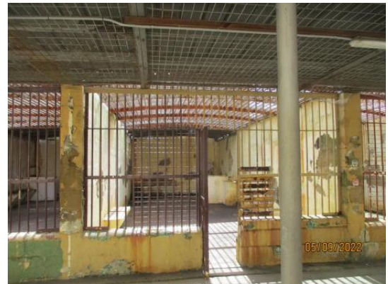
Figure 34 Interior of a typical yard
