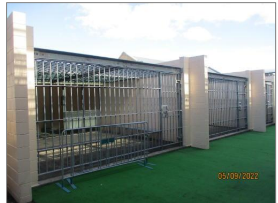
Figure 36 View of the Eastern Extension. Shows the new Yards in the foreground and the cell block behind.
