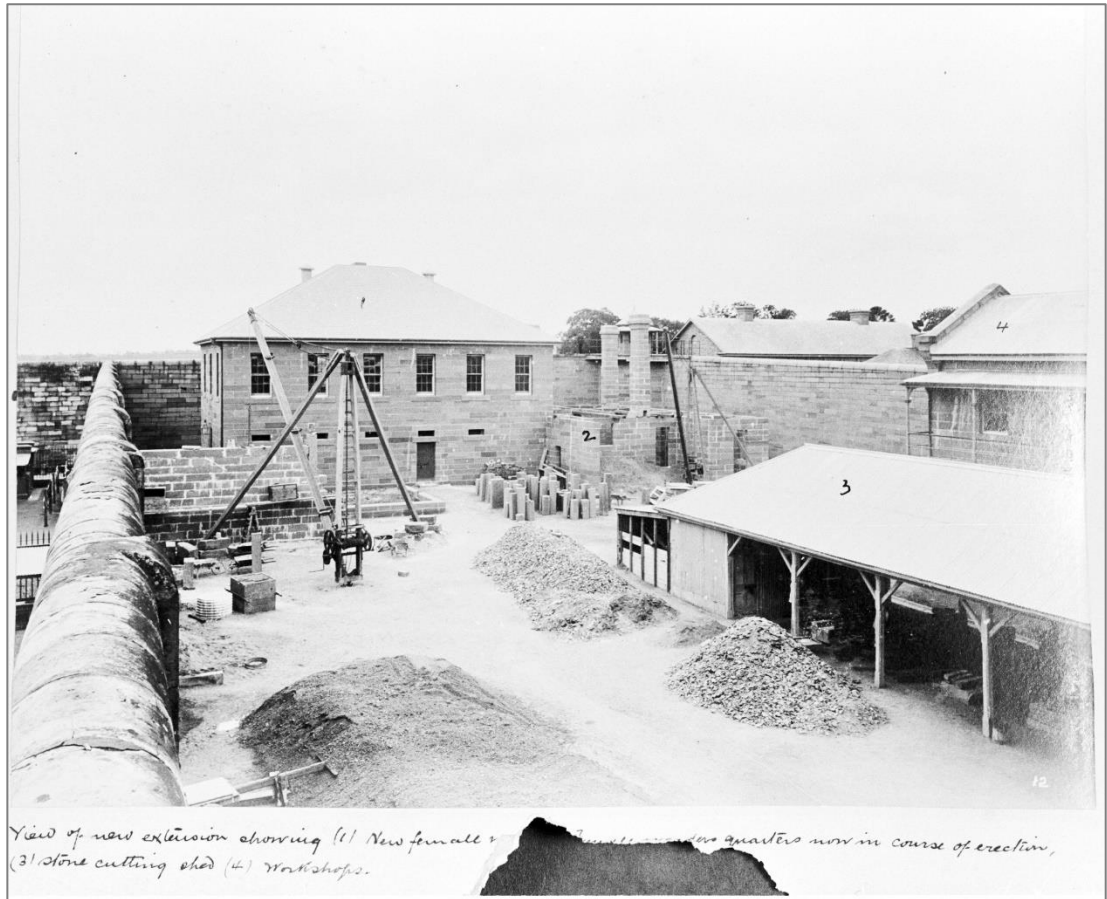
Figure 17 Eastern Extension 1: Female Wing; 2: Female warders' quarters in course of erection; 3: stone cutting shed; 4: workshops, c. 1897.
