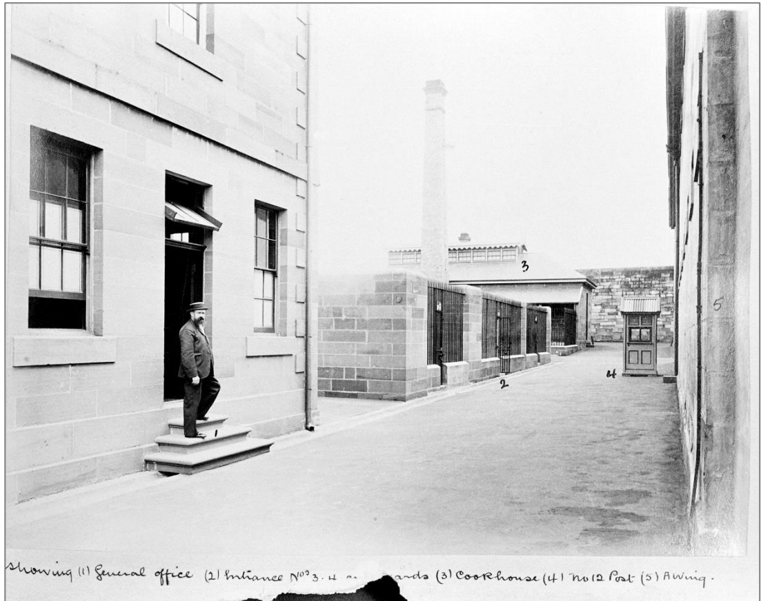
Figure 59 View looking north-east between Asset No's 005 and 009. This photograph shows an early configuration of the special yards, with the Cookhouse in the background. The wall of the closest yard in the c1897 photograph has been blocked in and an opening created on the north-western side. An infill wall at the end of this space and lightweight shelter-type structures built over this space detract from the appreciation of this area.
