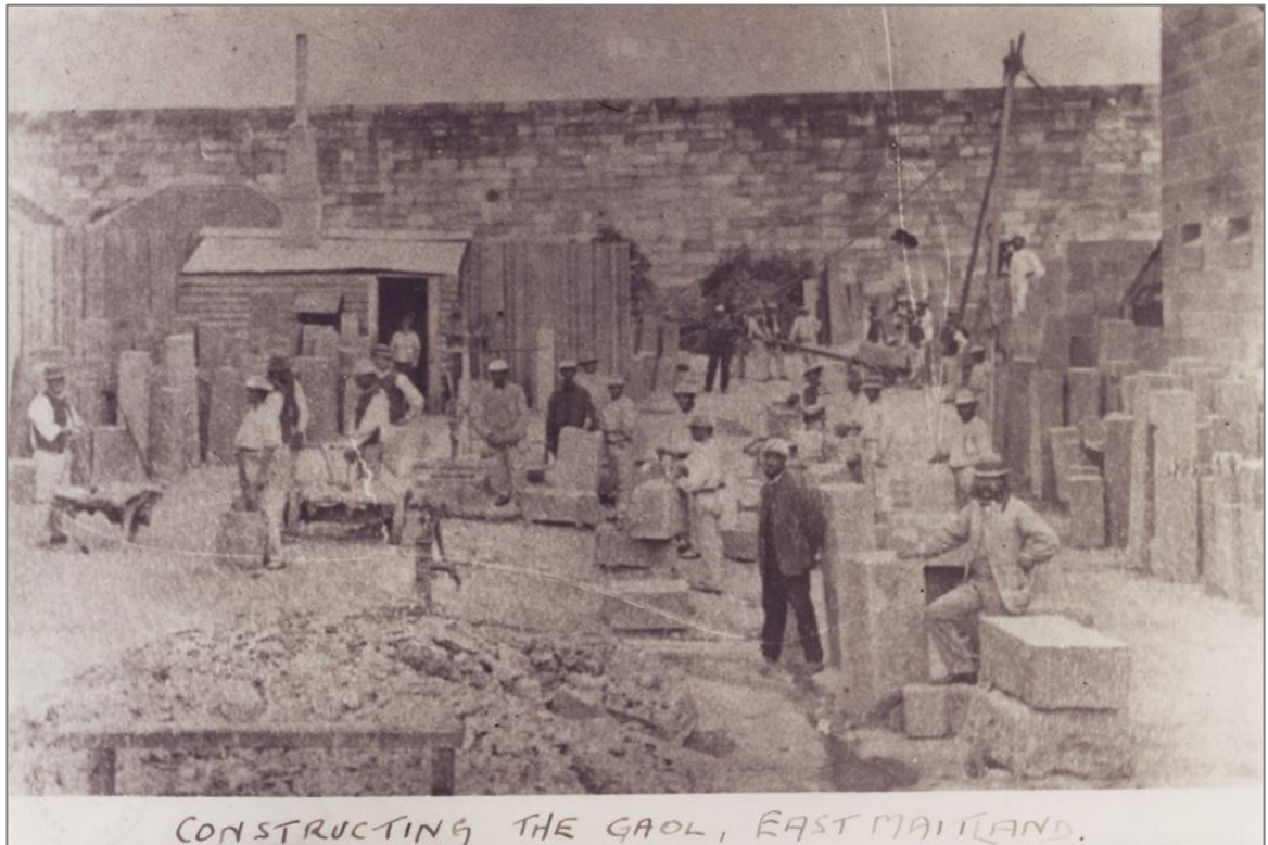
Figure 39: Constructing the Gaol
