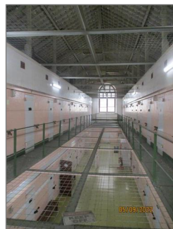
Figure 12 Interior of A Wing
