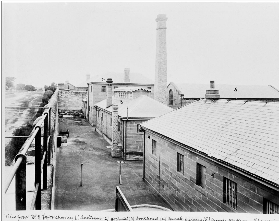
Figure 58 View from North Tower looking towards Asset No's 013 and 009. This photograph clearly shows the two buildings: the Cookhouse (3) and the Female Surgery/Workroom buildings (4) that were demolished to provide an open area. The Bathroom and Hospital (2) have been modified to create the present Kitchen Block.
