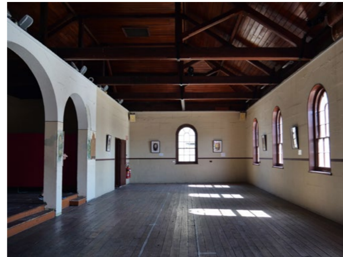
Plinths located in room under beams.
