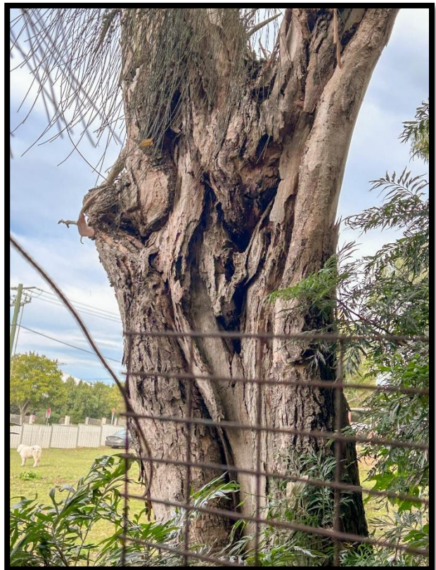
Decay in the trunk of the larger neighbouring tree.
