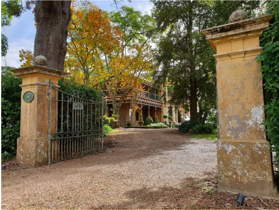
Figure 10: Anambah House gated entrance
