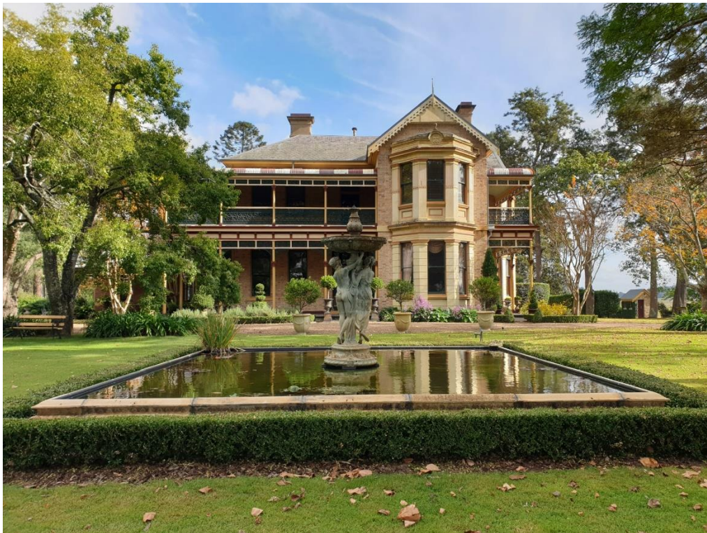
Figure 9: Eastern façade and main entrance of Anambah House
