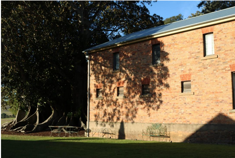
Figure 12: Western façade of the stables
