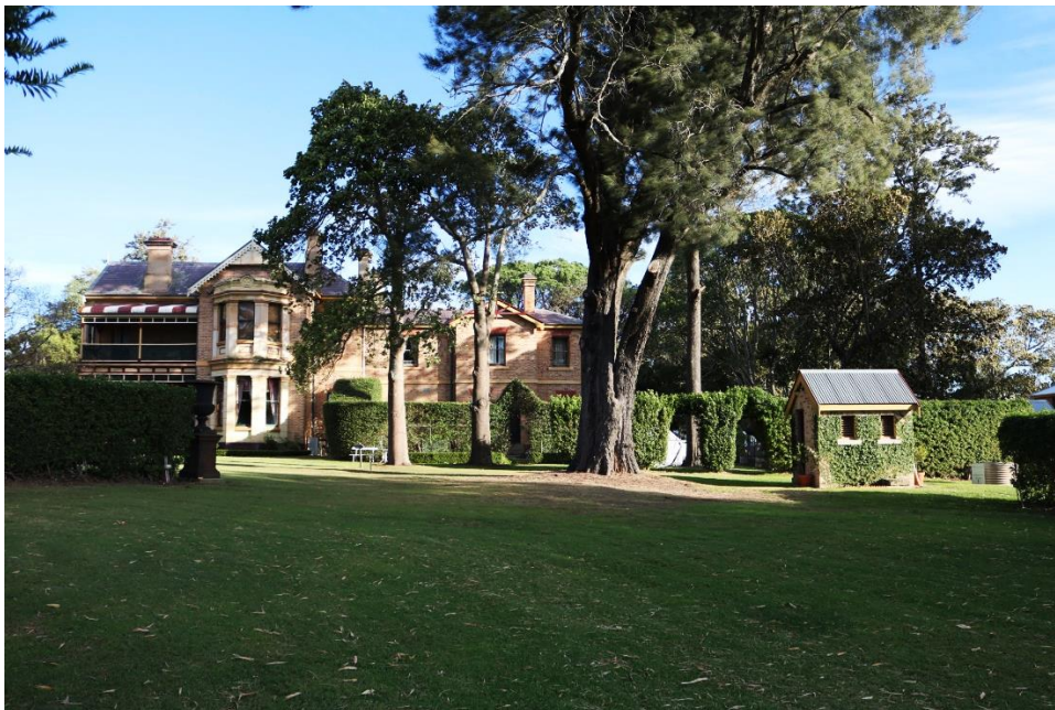
Figure 13: Northern elevation of Anambah house and outhouses
