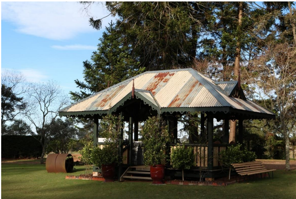
Figure 14: image of the tennis court pergola, taken on 9/06/2023
