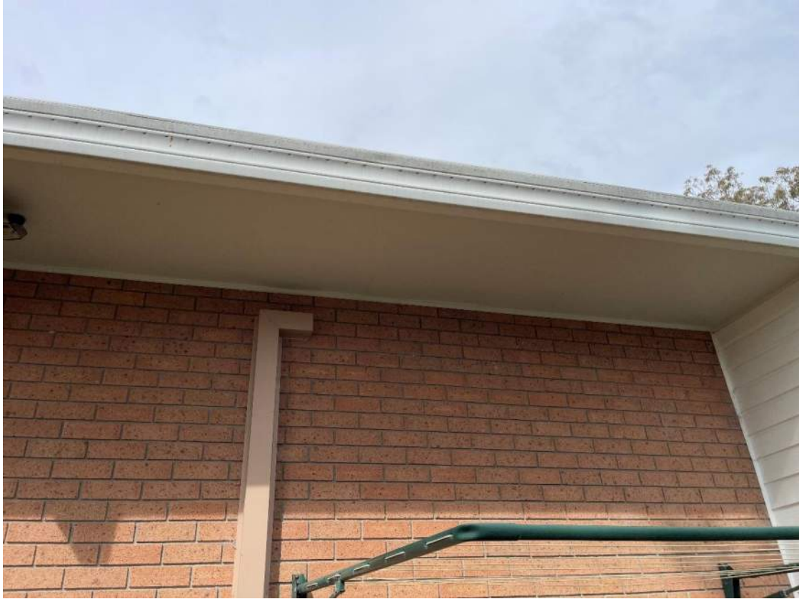
Photograph 9: View of the eaves of the residential dwelling, facing south. 14/08/2023.
