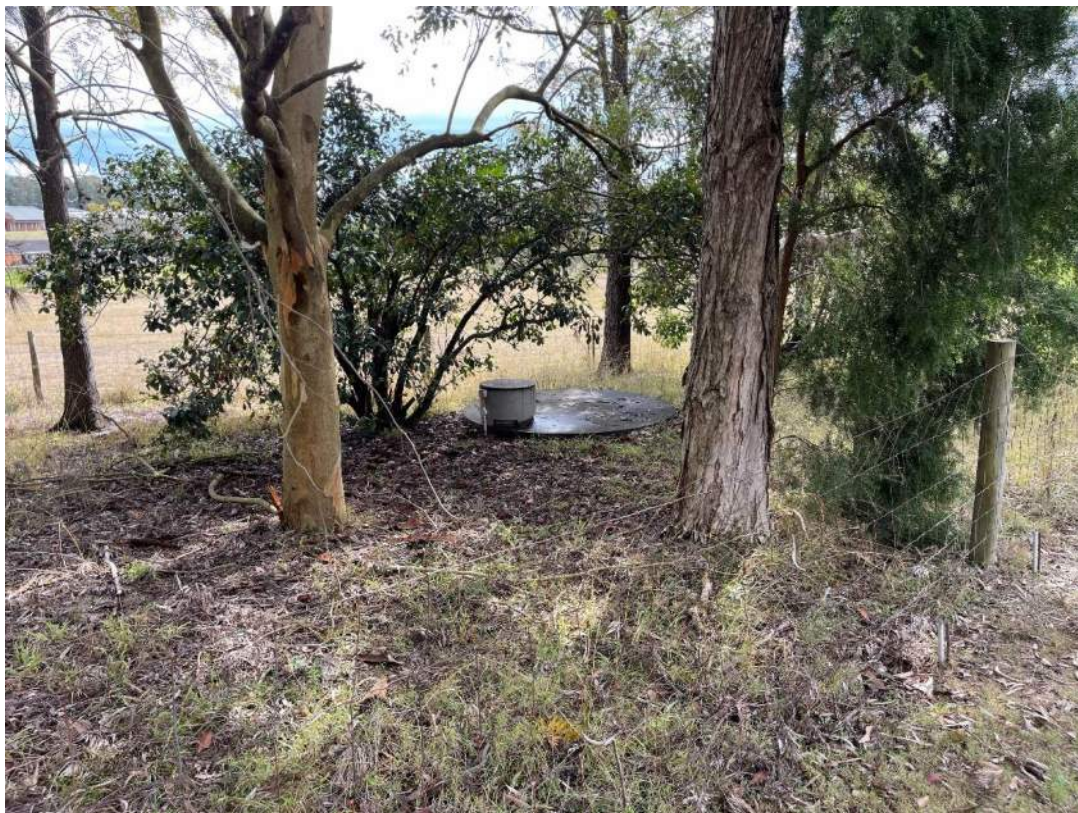
Photograph 8: View of septic tank north of the dwelling, facing north. 14/08/2023.
