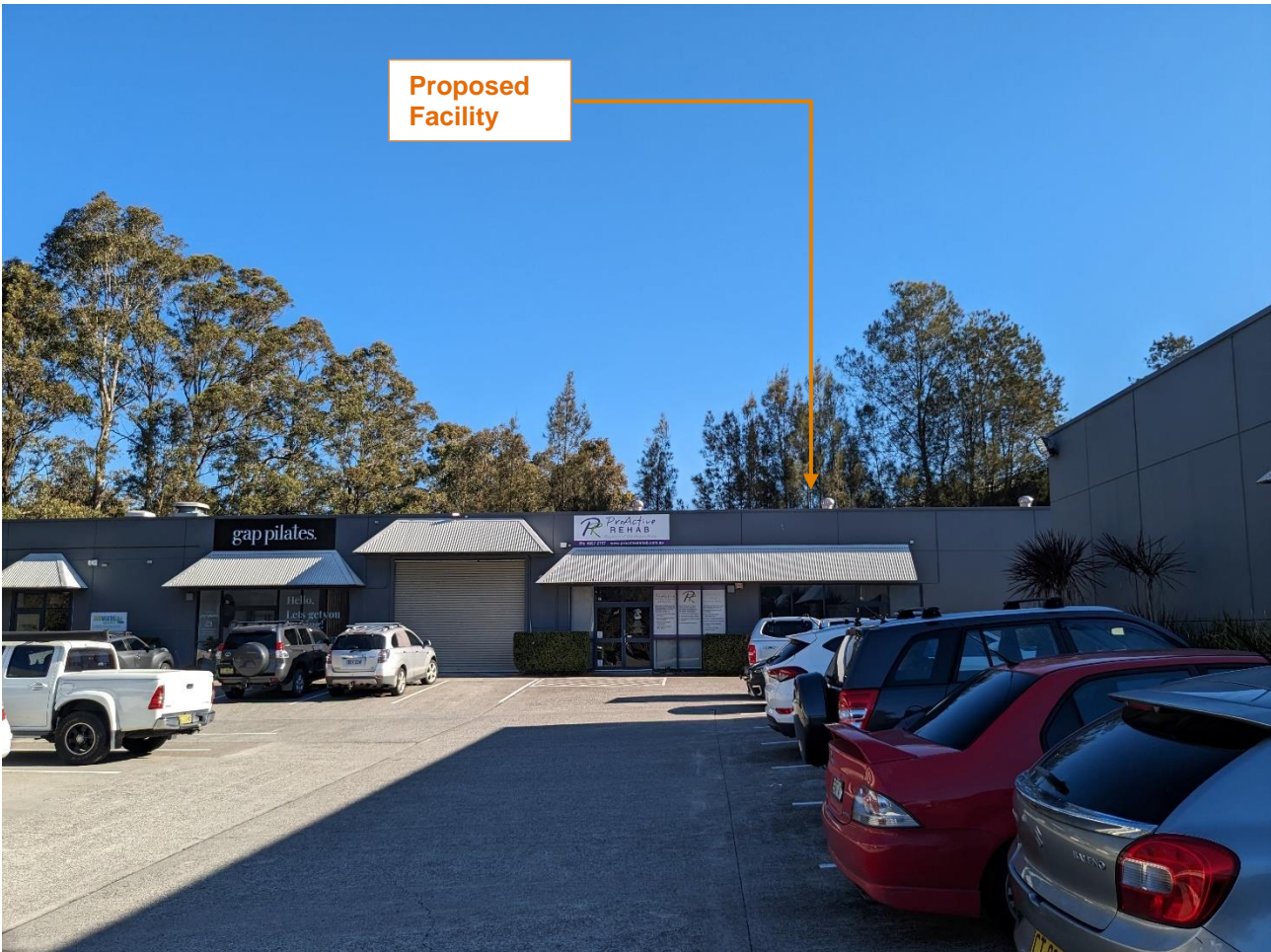
Figure 7: View looking south west towards the proposal from Molly Morgan Drive. The top of the monopole and antennas will be visible from Molly Morgan Drive
