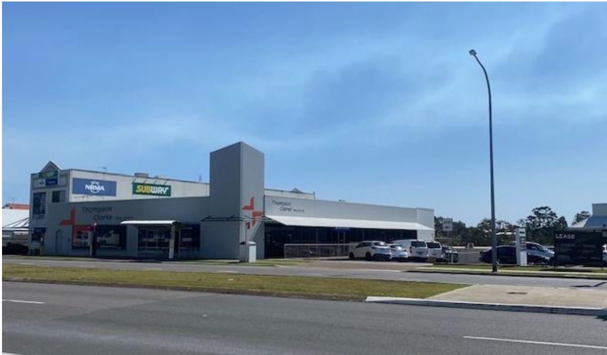
Figure 3.2 – Existing commercial building and existing entry driveway into the site from Mitchell Drive East Maitland
