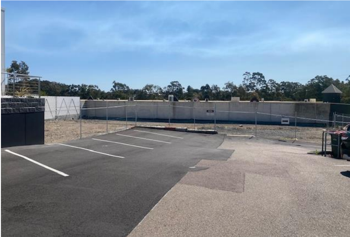
Figure 3.4 – Existing site previously occupied by Hit and Dip squash courts and gymnasium and a Chinese restaurant which have since been demolished.
