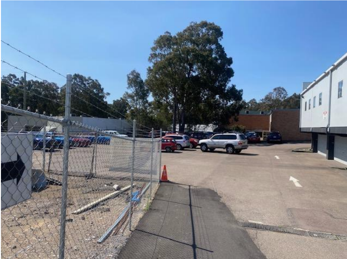
Figure 3.6 – Existing car park at rear of site
