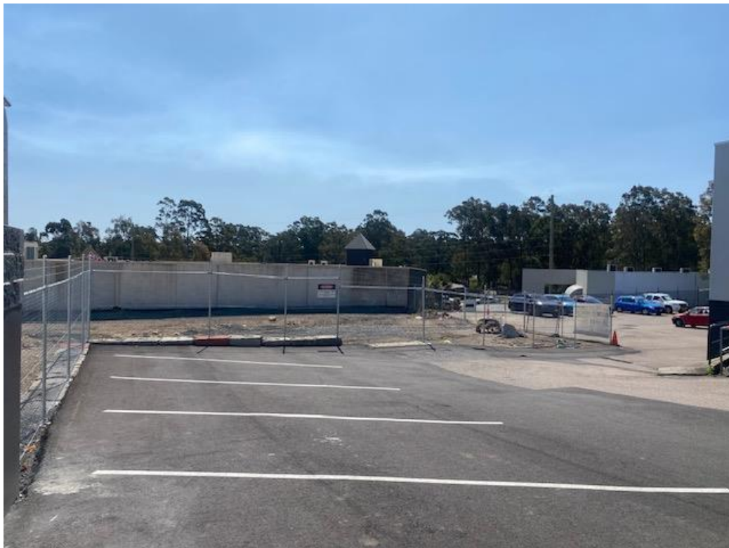
Figure 3.5 – Existing rear of site
