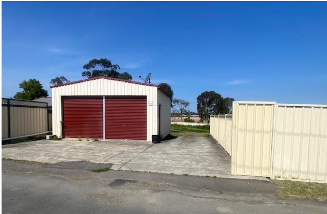
Figure 7 – Photo of existing double garage to be demolished
