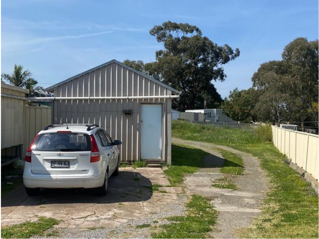
Figure 6 – Photo of existing shed to be demolished and rear yard at 52 Glenroy St Thornton
