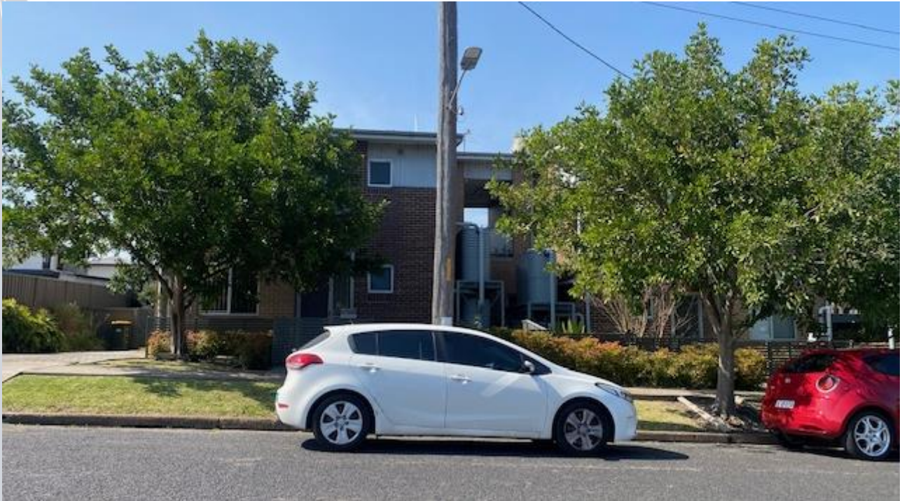
Figure 11 – Photo of recently constructed units on Glenroy Street
