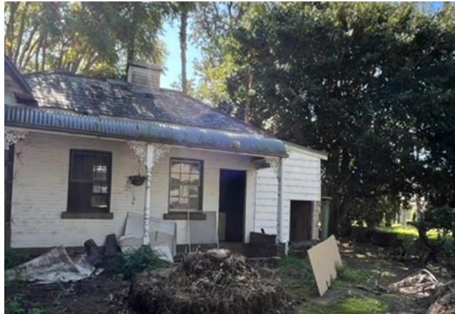
Photo 3: Presumably former servants' quarters to be converted to guest room
