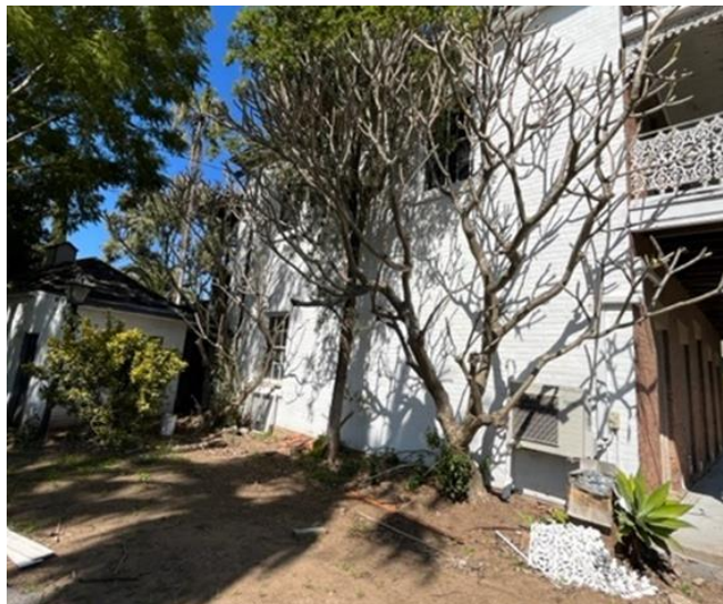
Photo 4: Northern façade of Hannan House
