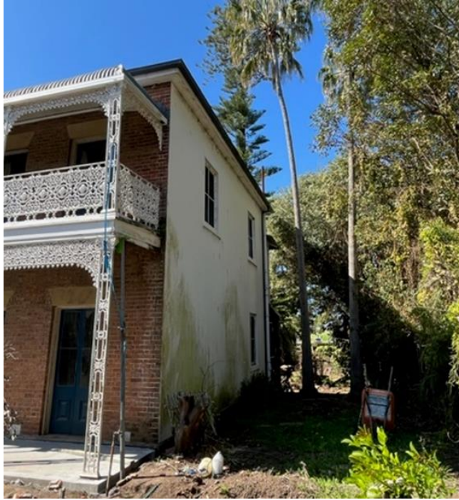
Photo 5: Southern façade of Hannan House
