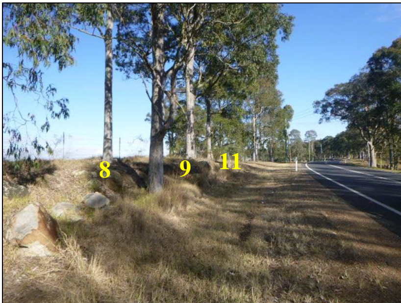
Photo 2 – Road widening not expected to encroach into TPZ
