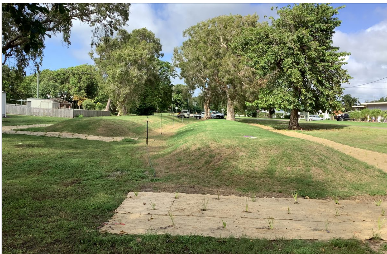
Figure 10.3 – Two newly commissioned Engineered Mounds at a Council owned Caravan Park
