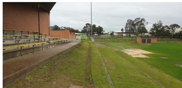
Photograph 8: From near centre of eastern boundary of site, facing north.
