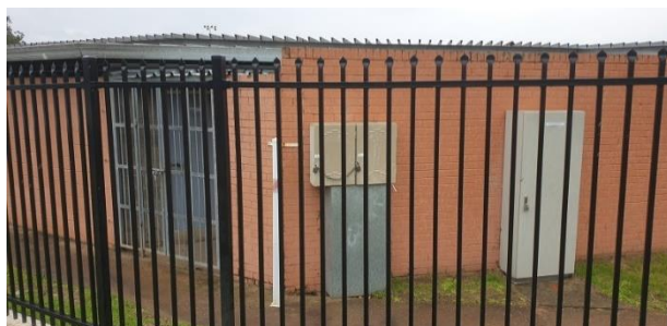
Photograph 3: From near centre of western boundary of site, facing east.
