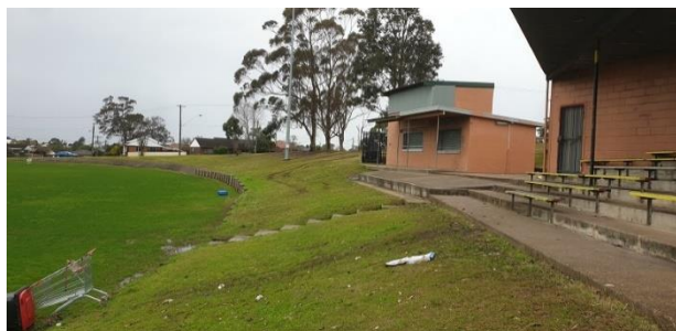
Photograph 7: From near centre of eastern boundary of site, facing south.
