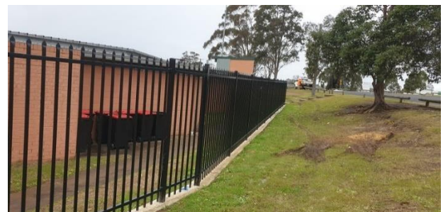
Photograph 4: From near centre of western boundary of site, facing southeast.
