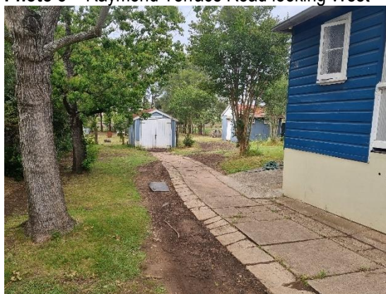
Photo 5 – Existing driveway, garage and shed at 39 Raymond Terrace Road. Sheds and driveway to be demolished
