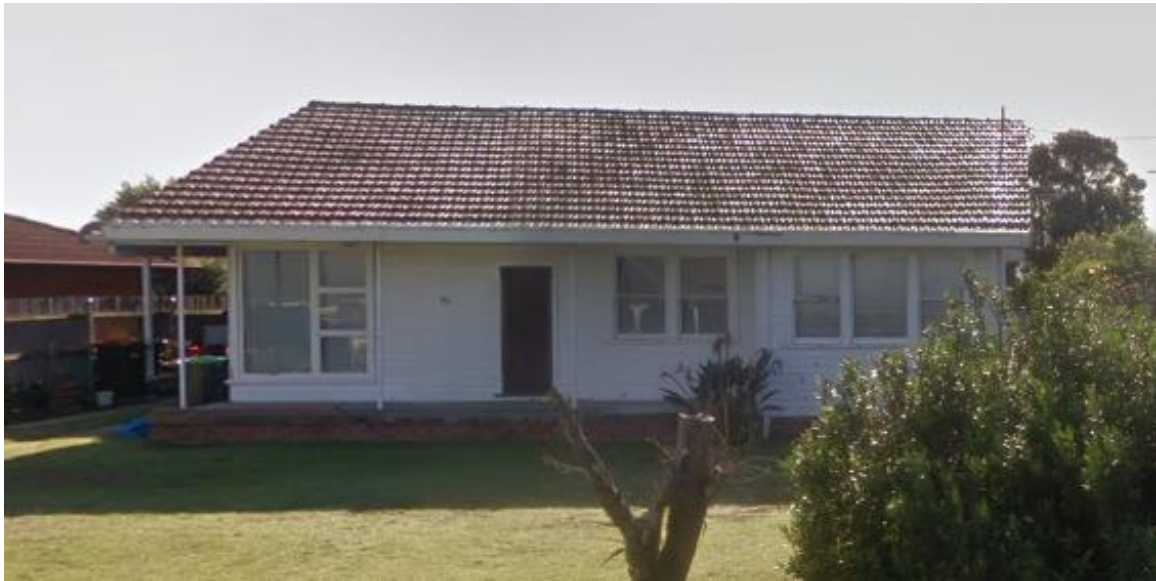
Photo 1: Dwelling to be demolished
