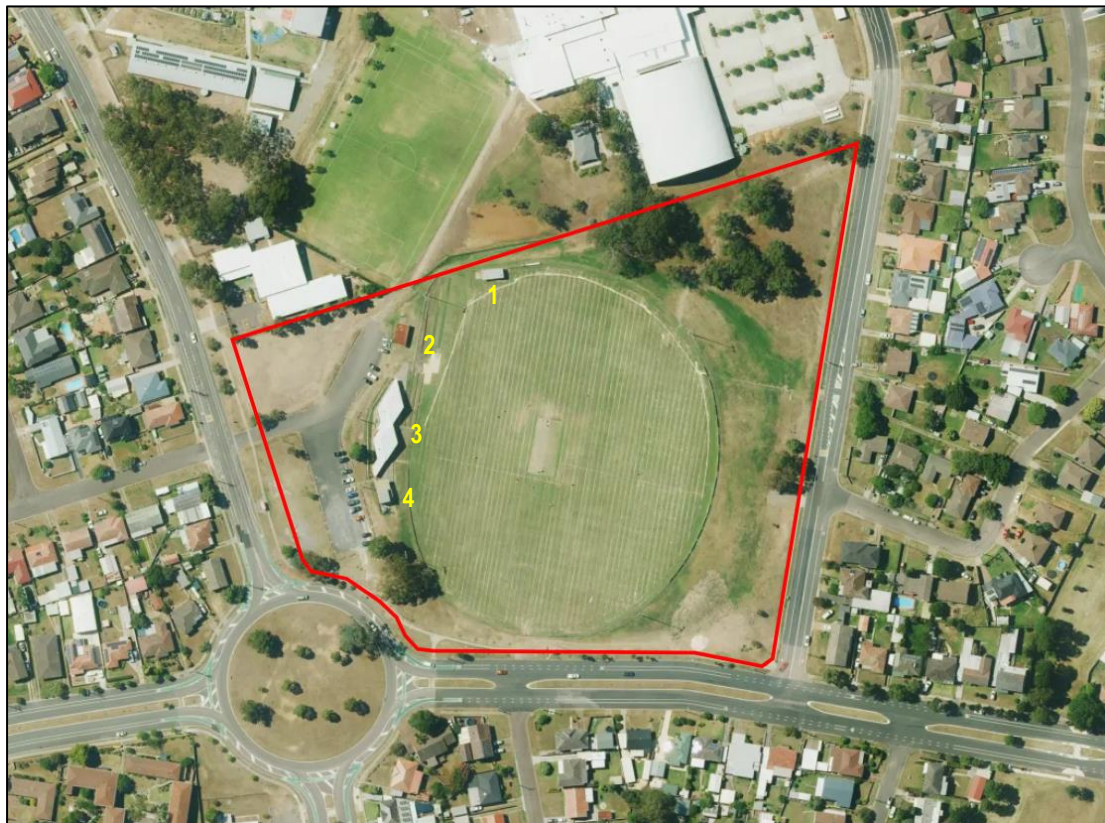
Figure 1: Aerial overview. Site outlined in red (aerial © Aerometrex 2023)
