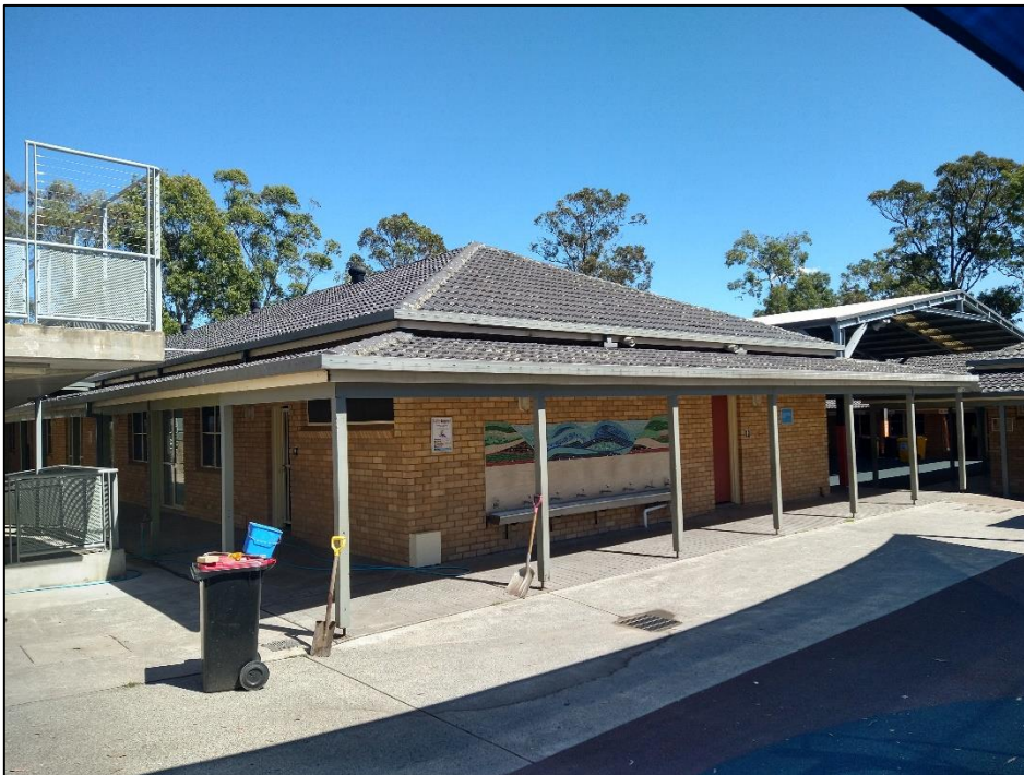
Figure 4: Rear of Block C, looking north-west. COLA beyond.
