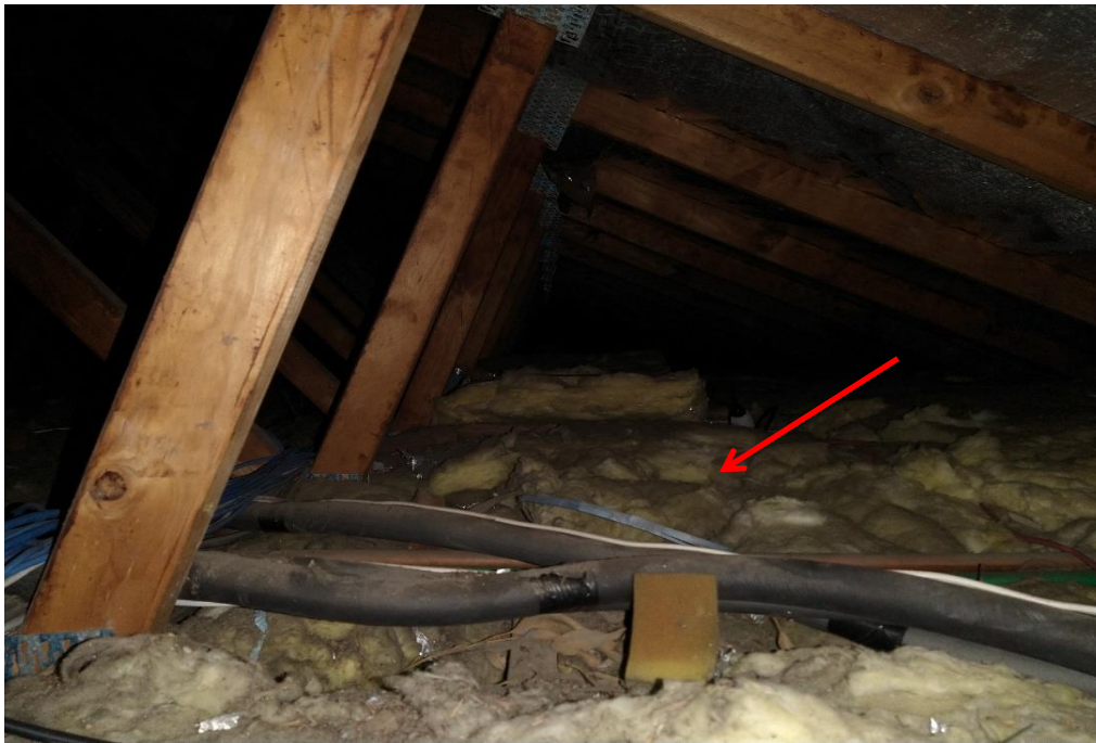
Photograph 16: Block B, interior, ceiling / roof space, insulation, SMF identified visually
