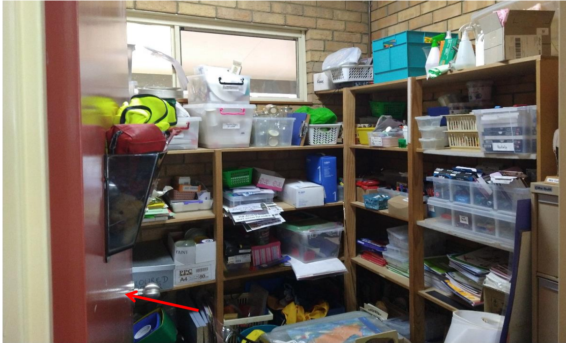
Photograph 1: Block B, B1 - interior, internal door, red, grey, blue layered paint, non-lead paint ( \leq 0.1\% lead w/w)
