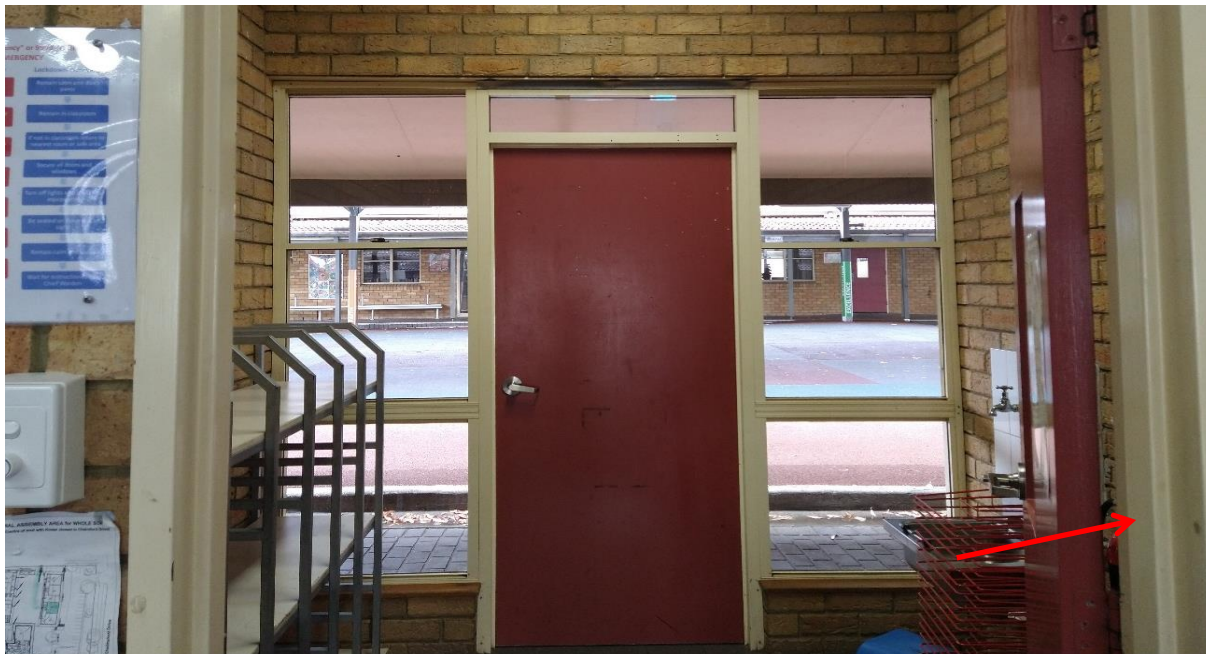
Photograph 4: Block B, B4 - interior, internal door frame, cream paint, non-lead paint ( \leq 0.1\% lead w/w)
