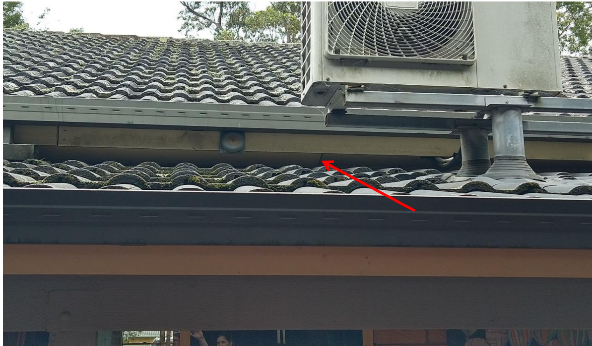
Photograph 11: Block B, exterior, eave lining, fibro sheeting, suspected non-asbestos
