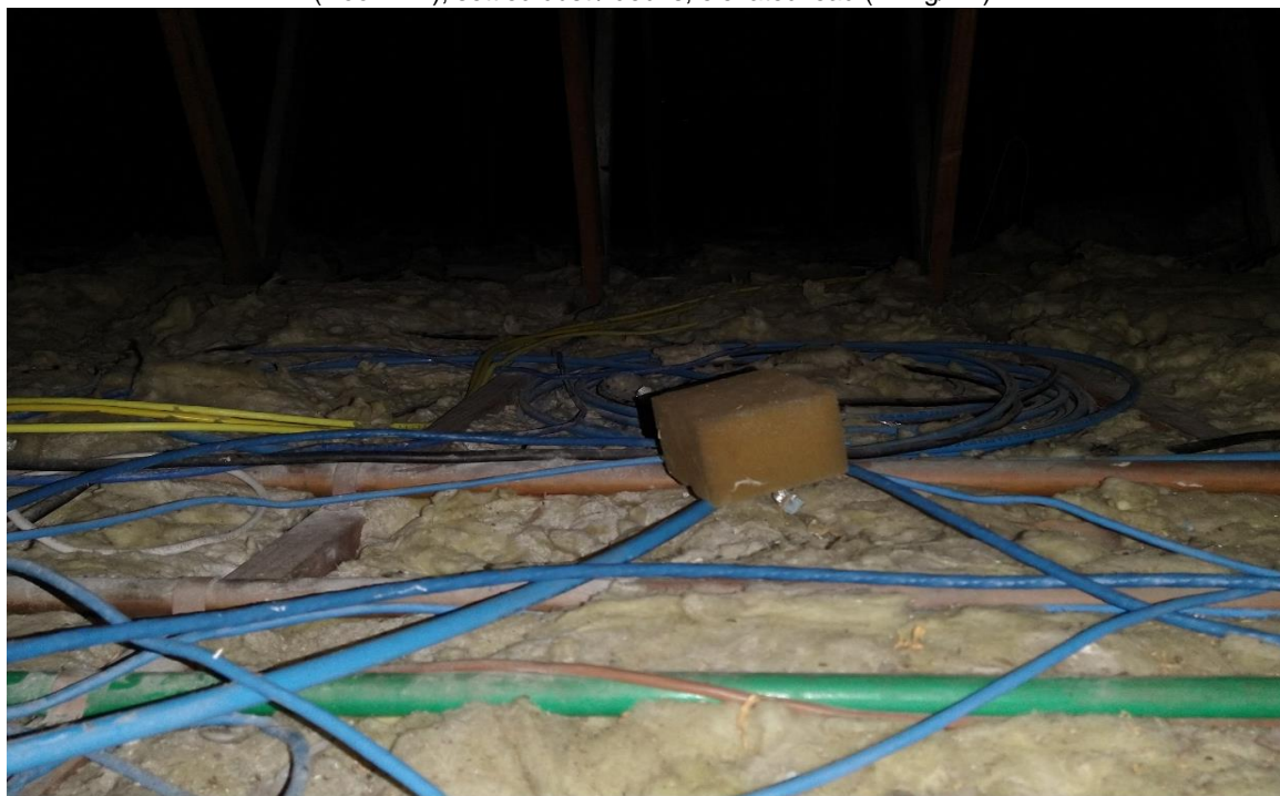
Photograph 6: Block B, B2 - interior, ceiling / roof space (Room B2), settled dust / debris, elevated lead (11mg/m2)
