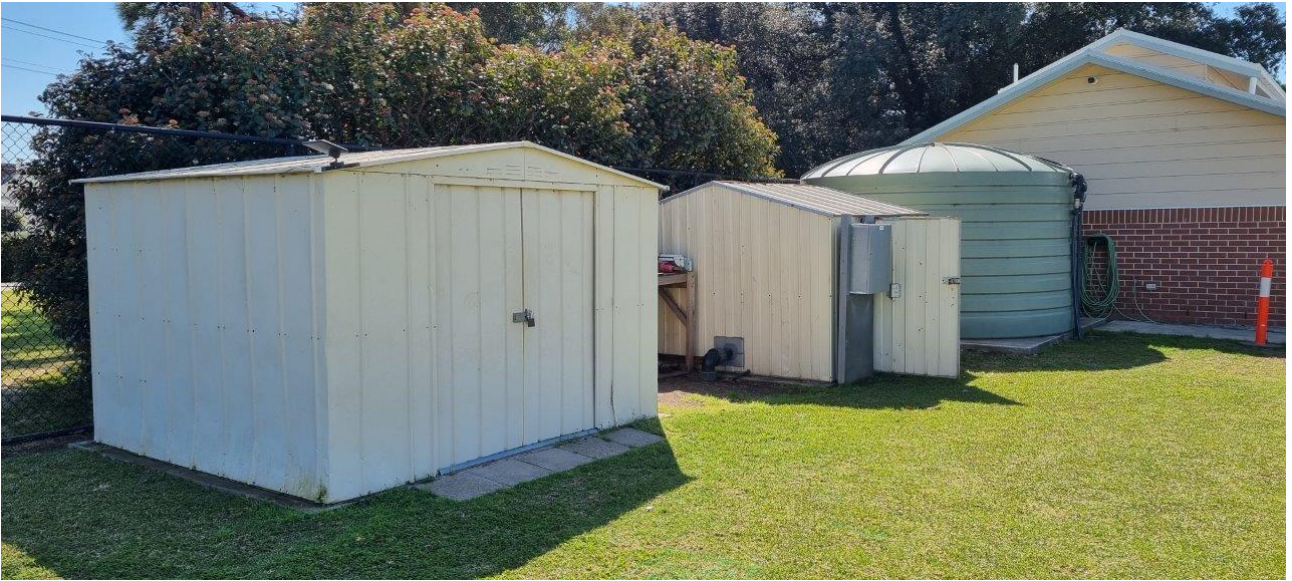
Figure 2 – Existing Maitland Hockey Club facilities, rainwater tank and sheds (sheds to be replaced).
