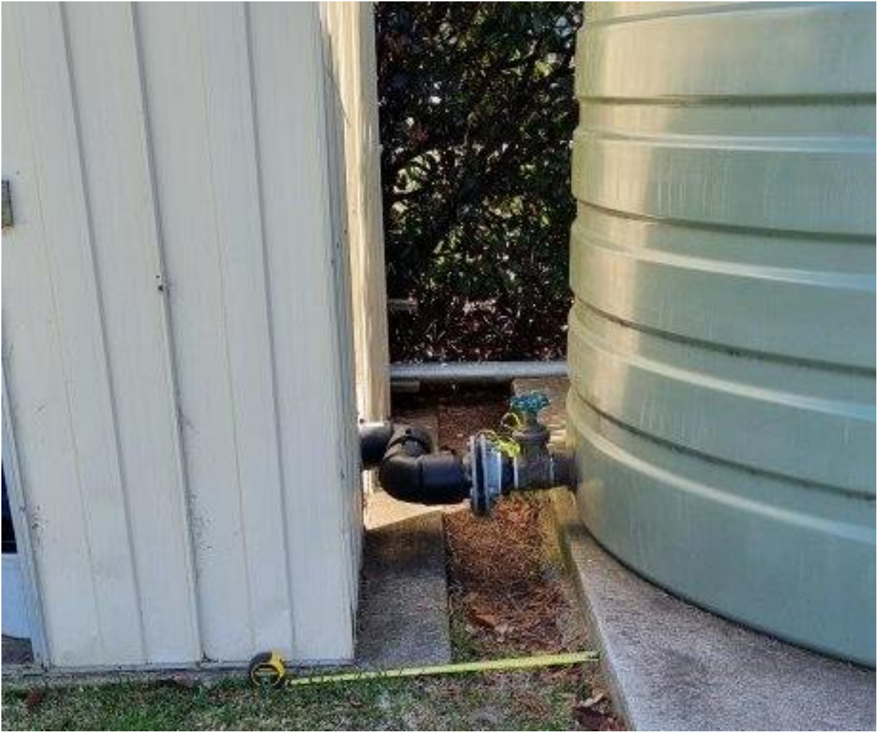
Figure 4 – Existing rainwater tank, pump (in shed) and connections to be retained.
