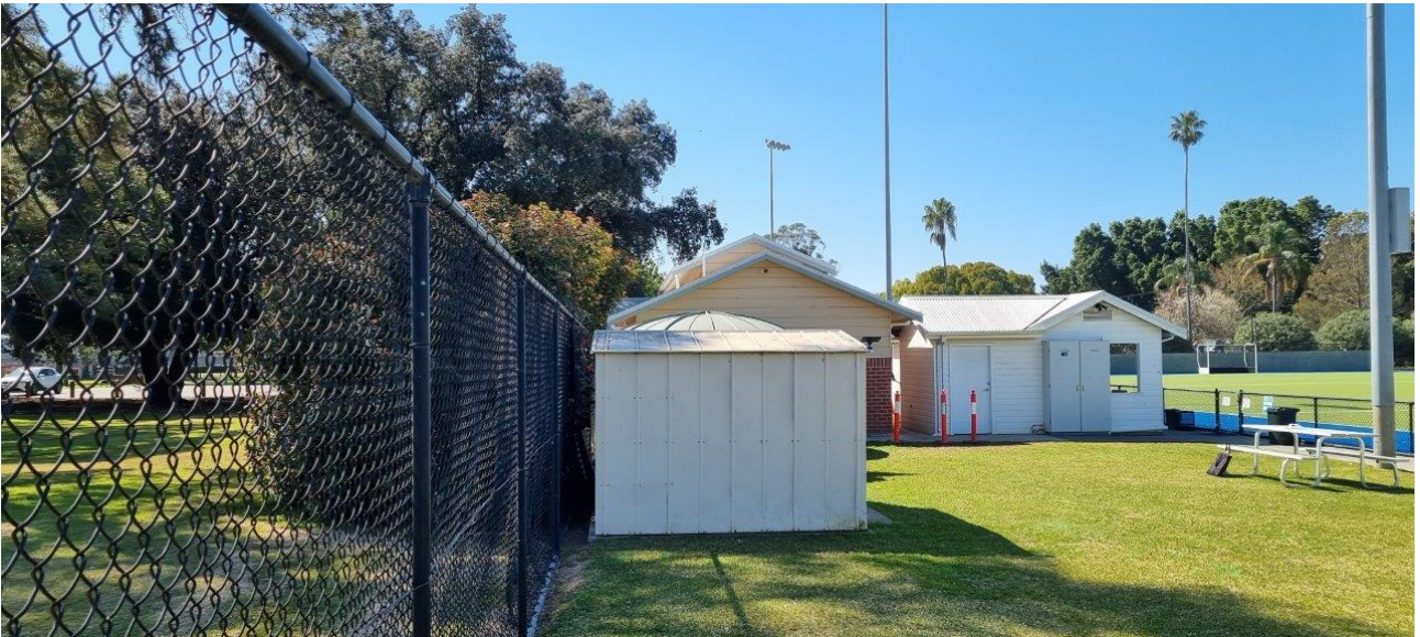
Figure 3 – Existing sheds to be replaced, the proposal retains the existing fence offset.
