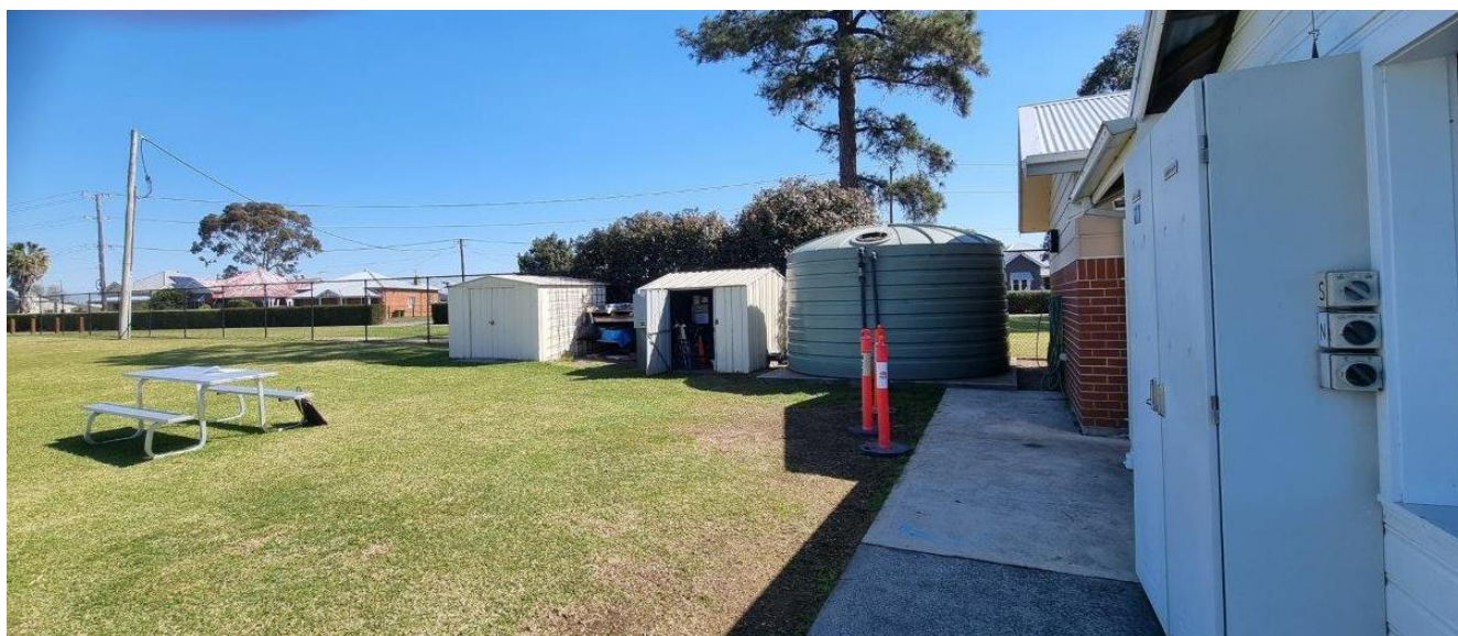
Figure 1 – Existing Maitland Hockey Club facilities, rainwater tank and existing sheds (sheds to be replaced).
