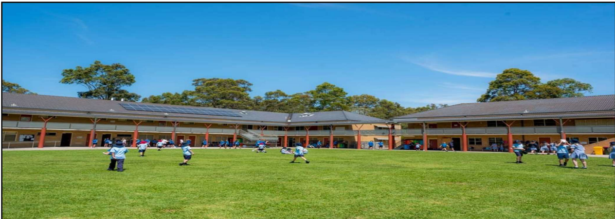
FIGURE 5- EXISTING SCHOOL IMPROVEMENTS
