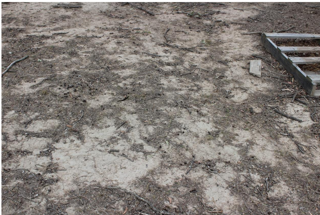
Plate 2. Example of erosion to basal clay. (Source: Heritage Now 2023)
