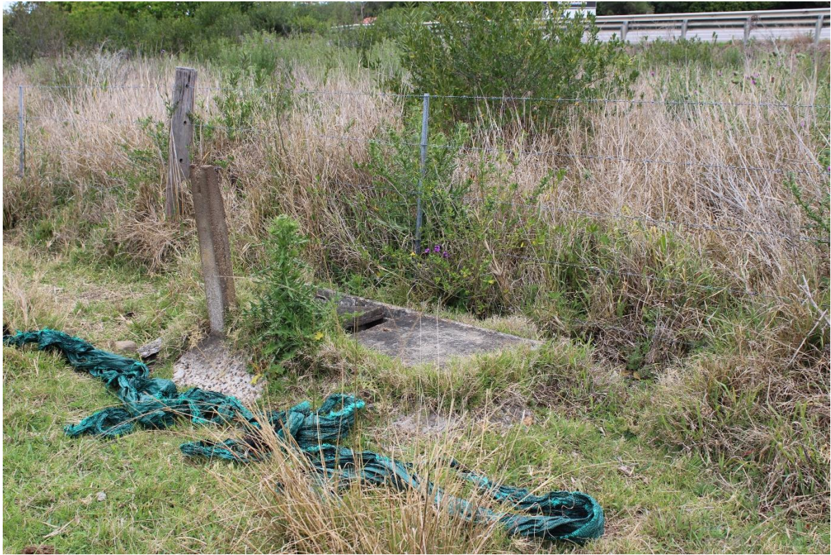
Plate 9. Evidence of water infrastructure along the southern boundary of the Project Area. (Source: Heritage Now 2023)
