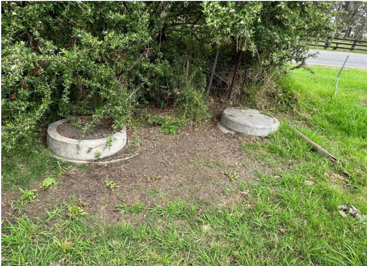
Photograph 40 - Sewer inspection holes in south western corner of site -10 River Road.
