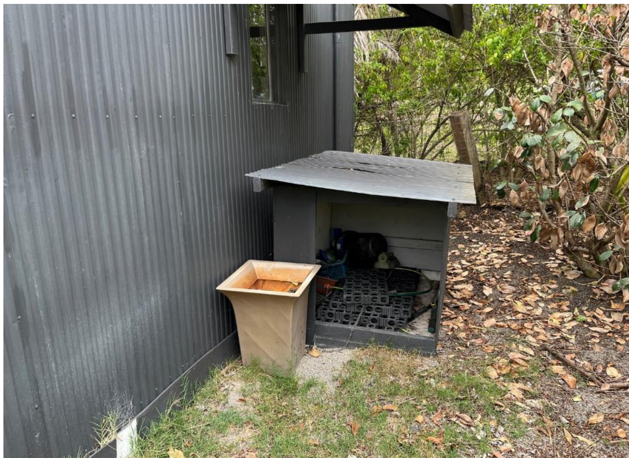
Photograph 54- Small pump shed / dog kennel on northern wall of Dwelling 3.
