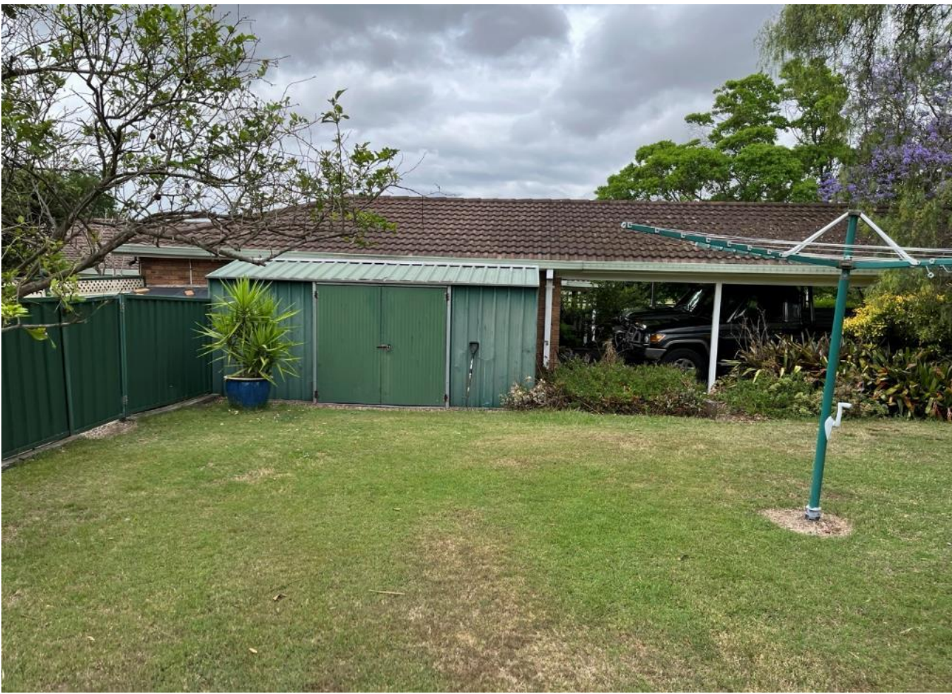
Photograph 11 - Carport 1, Shed 2 and Shed 1 west of Dwelling 1 - 10 River Road.
