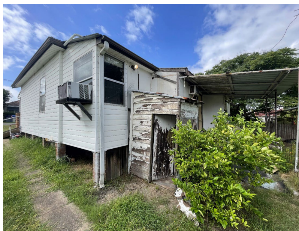
Photo 4: This image shows a highly weathered outhouse-like structure present in the central portion of the site adjacent to the house. This structure as well as the houses fascia and eaves paint are all very weathered and be a potential source for lead based paint contamination in AEC 3.
