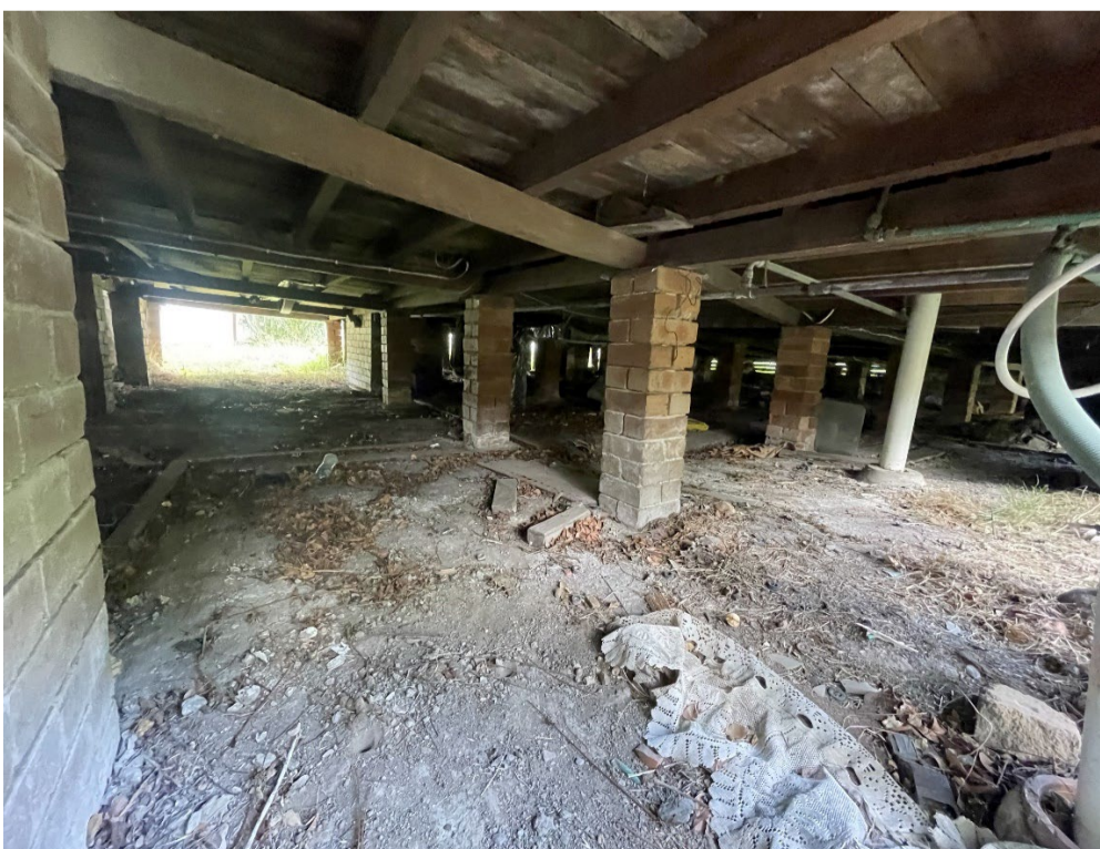
Photo 11: Overview of the subfloor at 63 Burg St, East Maitland.
