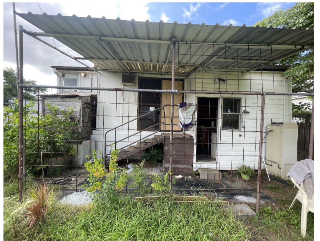
Photo 10: Overview showing the rear portion of the dwelling, looking southeast.
