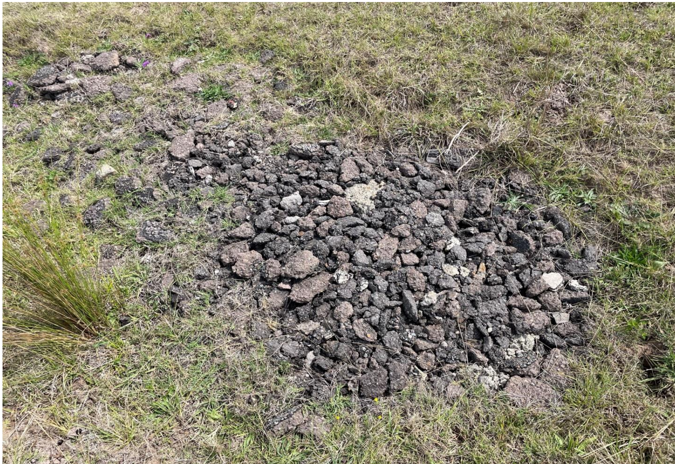
Photograph 29 - Asphalt in drainage line north of road crossing.
