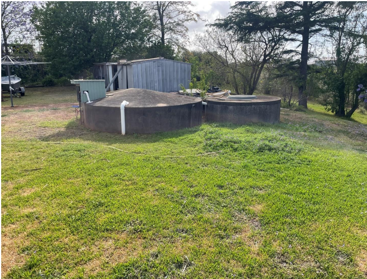
Photograph 17 - Water tanks located east of the dwelling.
