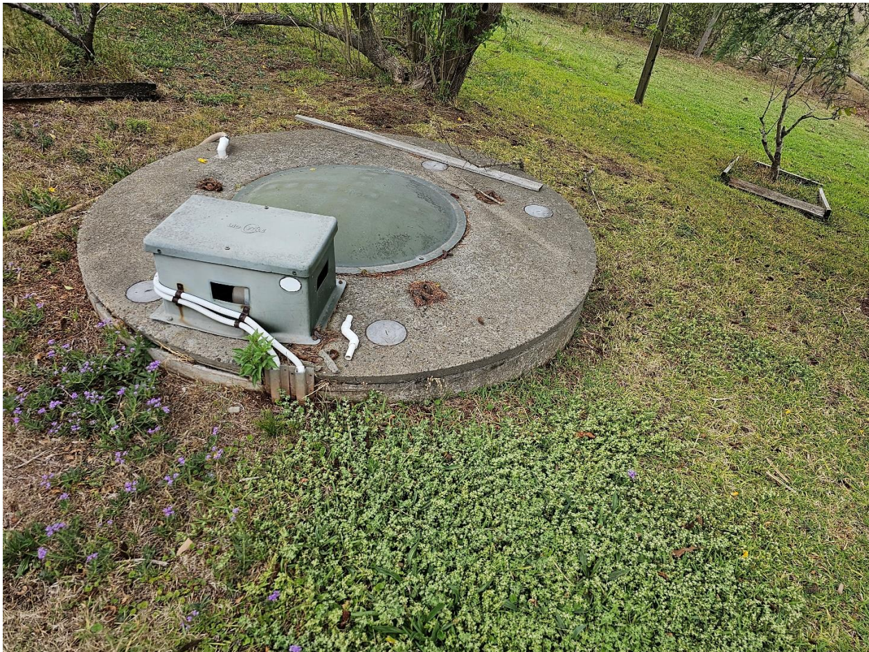
Photograph 18 - Septic tank located east of the dwelling.
