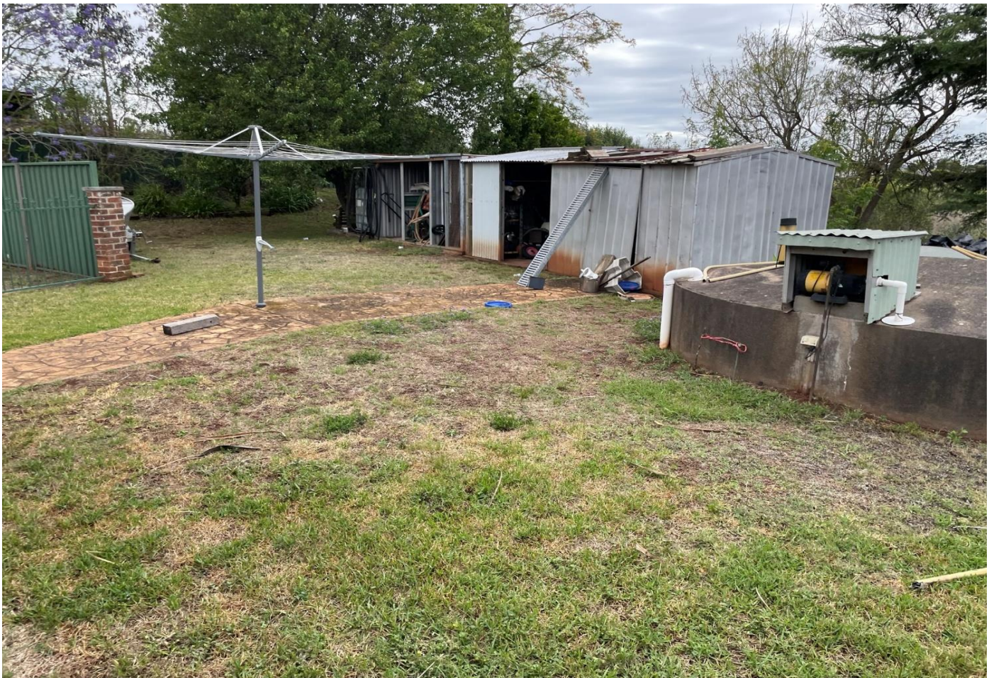
Photograph 5 - Shed 3 located east of the dwelling.
