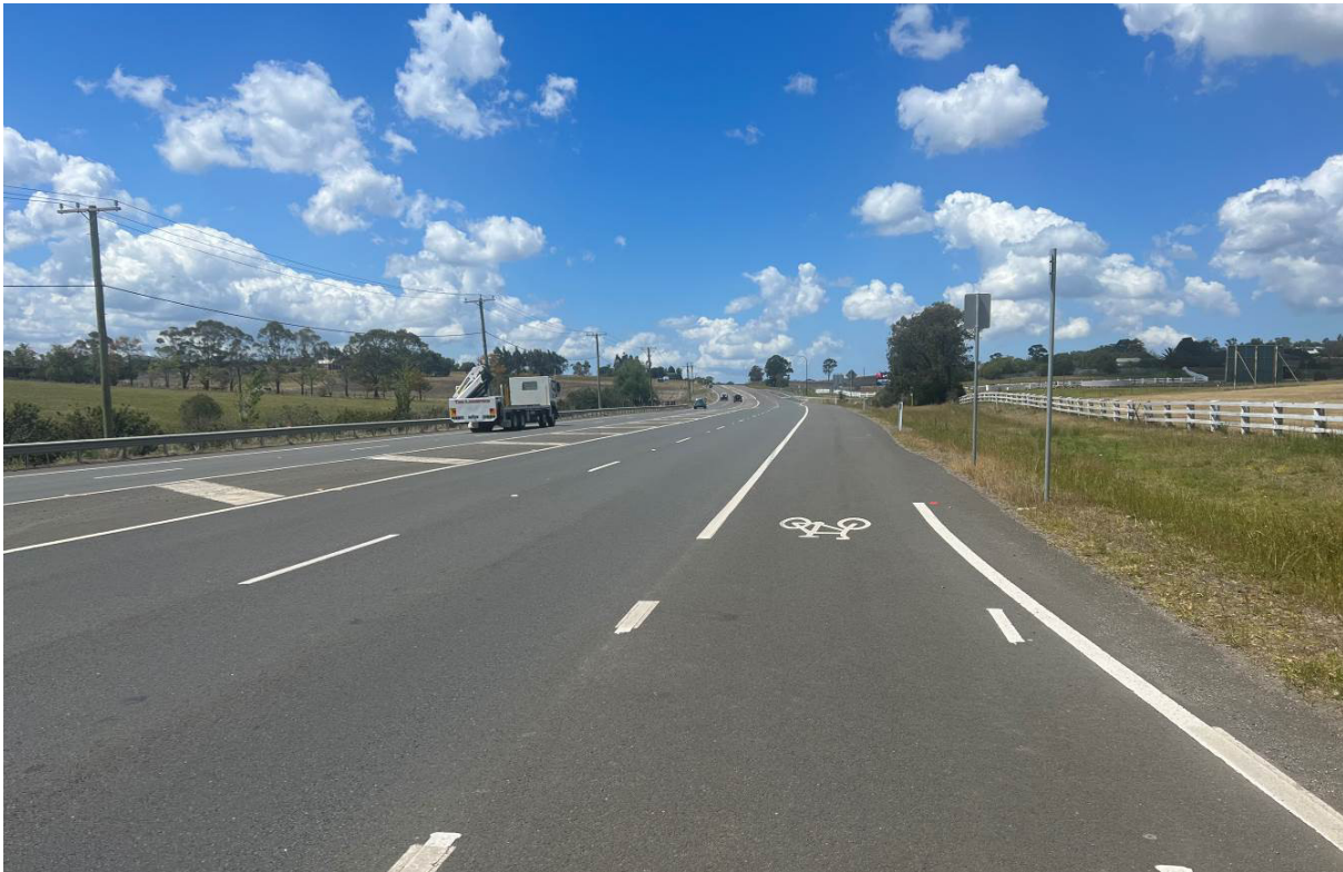
Photograph 3 – New England Highway near Wyndella Road intersection.
