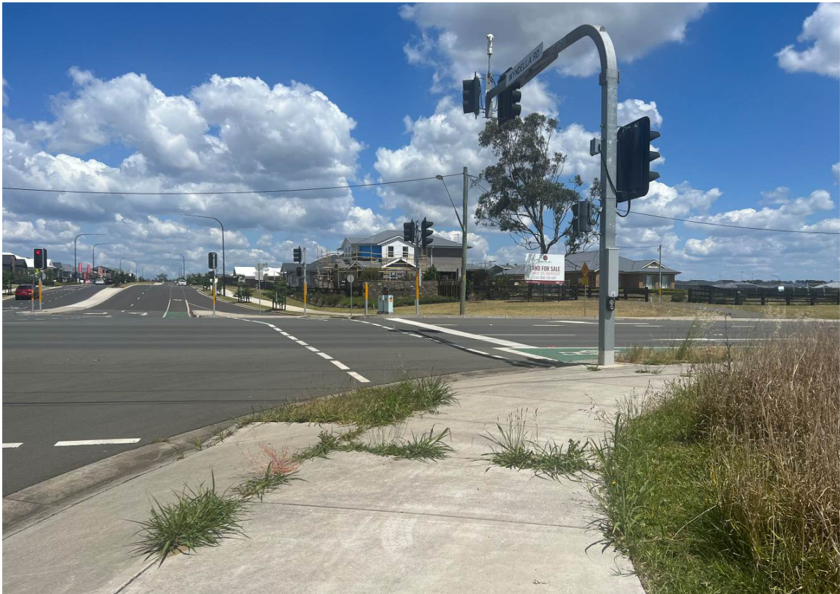
Photograph 7 – Pedestrian Crossing New England Highway / Wyndella Road signals.
