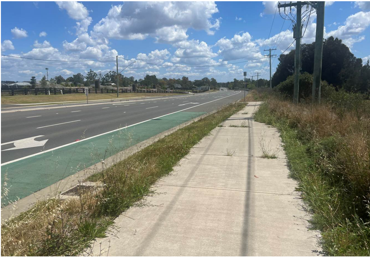
Photograph 6 – Bus Stops / Pathway New England Highway near Wyndella Road.
