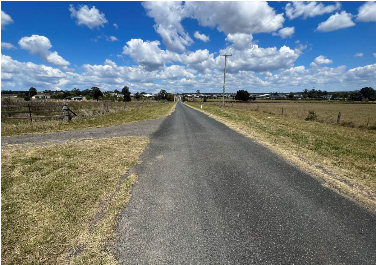
Photograph 4 – Wyndella Road south of site access.
