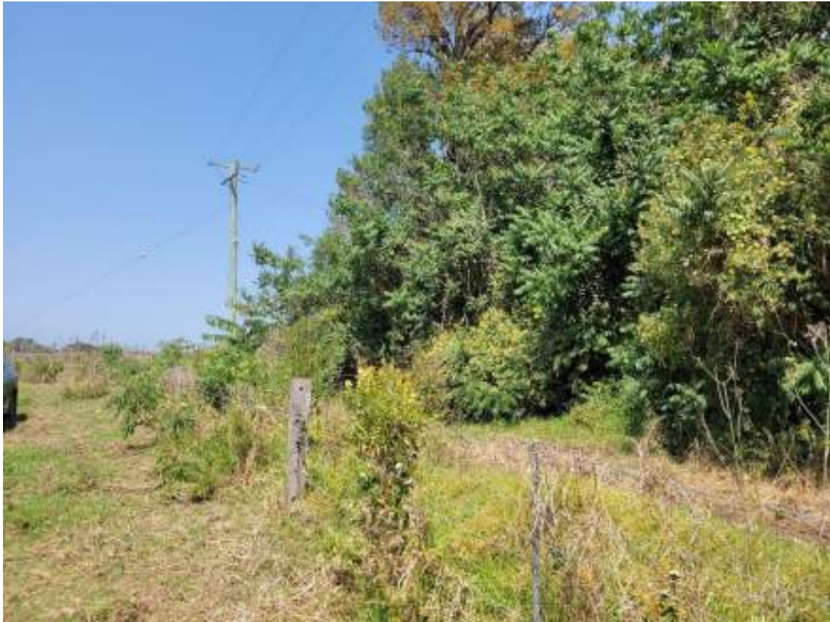
Plate 5-3. Non-native vegetation on western embankment. View from the north-east.
