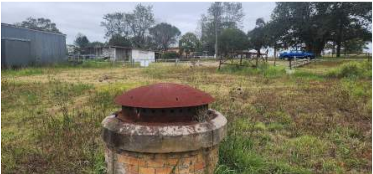
Figure 10 – (refer Figure 9 Image 07). Located within the Hunter Water easement, and located outside the area of projects works, this structure appears to be a remnant of the former intake pipeline to the Walka Water Works. Possibly an air vent and/or inspection portal. Further investigation is required to identify purpose and provenance. The presence of this remnant may provide an indication that some associated remnant works remain underground. MCC is in the process of acquiring the easement from Hunter Water. Historical records mention an inspection man hole with rickety iron ladder located east of the pump house.
