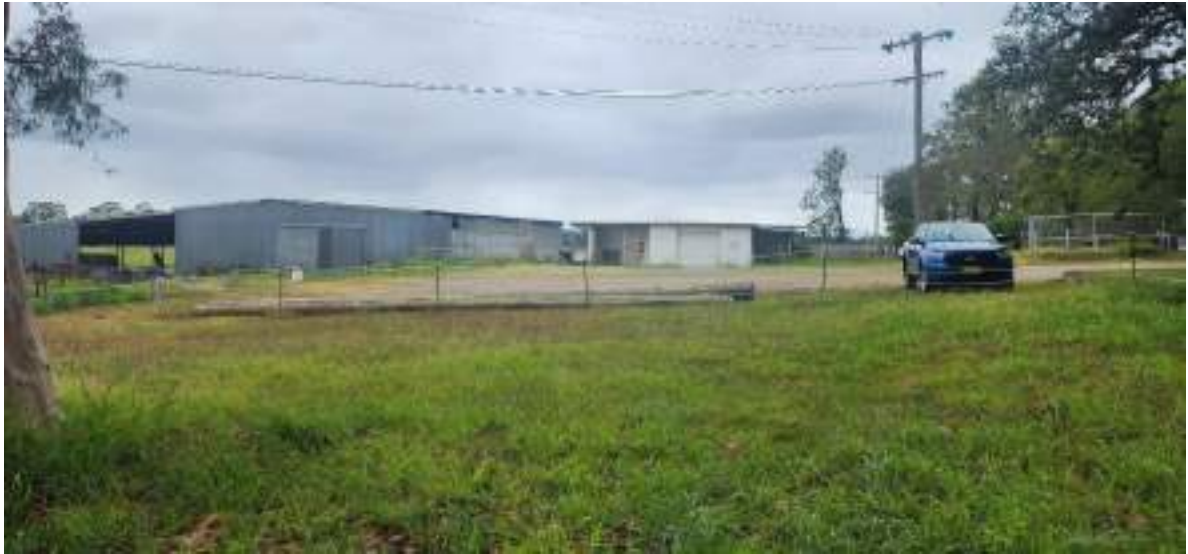
Figure 9 – (refer Figure 9 Image 03). Looking south along proposed line of re-alignment from the current Scobies Lane. The white building (former dairy building) is currently being demolished as it is within the proposed new alignment.
