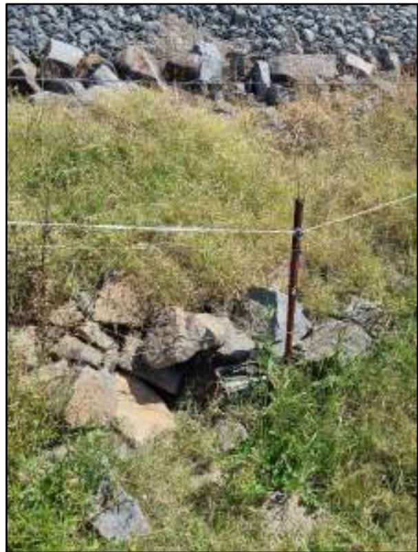
Figure 3-7 Blocked existing culvert below flood levee
